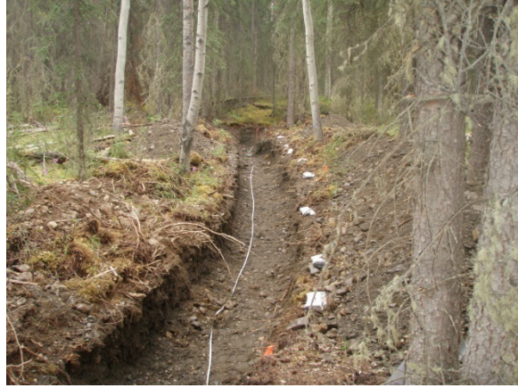
NC-TR-15-02, 2 nd pass to ~1m, looking south
