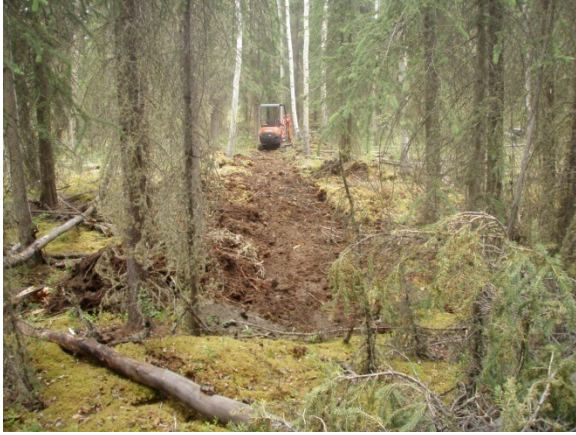
NC-TR-15-02, removal of the vegetative mat, looking north
