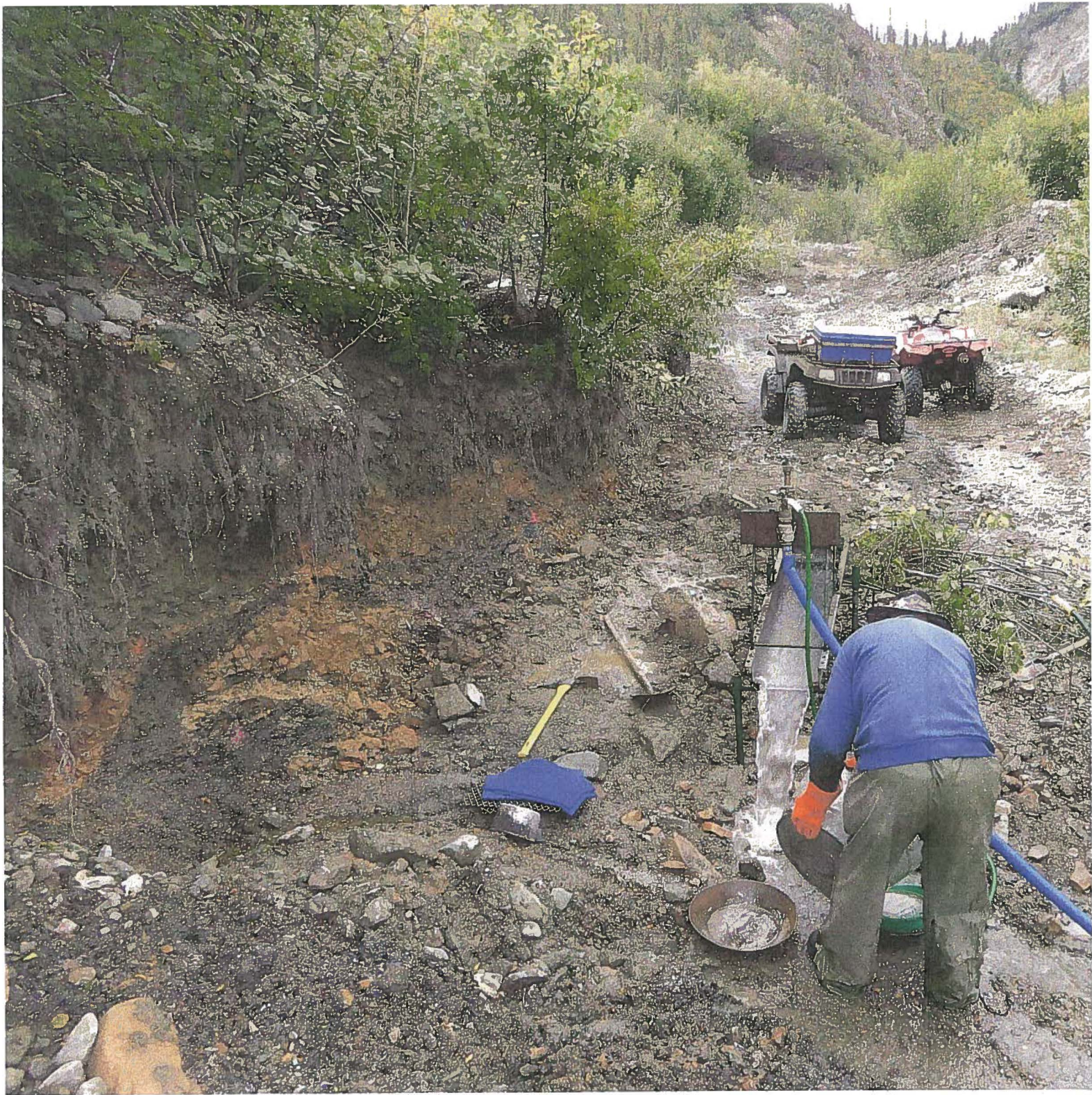
Photo 4: Trench 1 2019. Cleaning sample from sluice. On left is trench-bedrock face prepared for sampling. Looking south-upstream.to Lower Canyon
