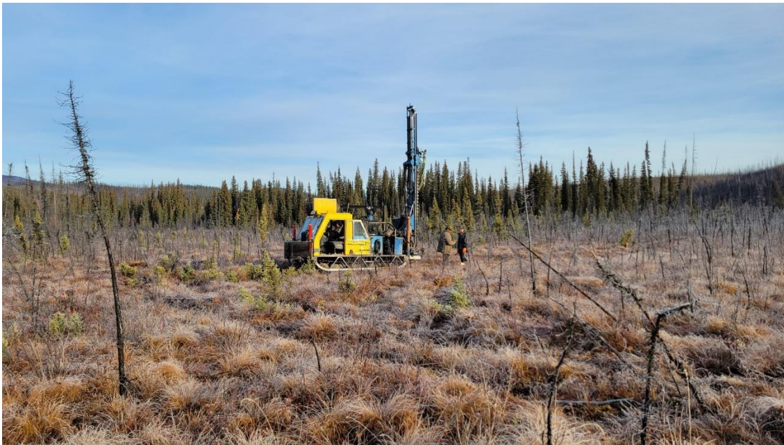
Figure 11.5: The Auger drill set up on a drill hole in the Twentymile creek.
