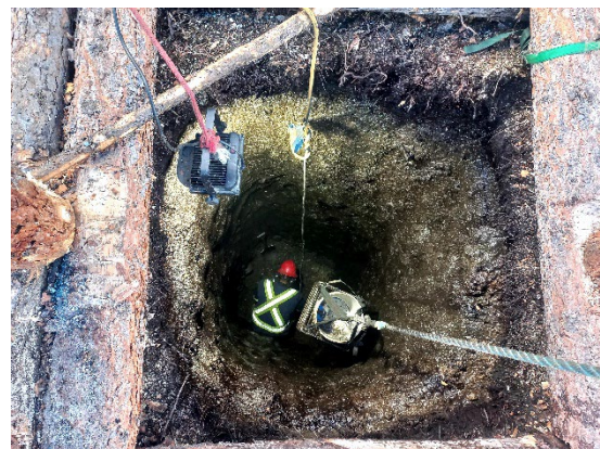
Figure 9: View down the shaft.
