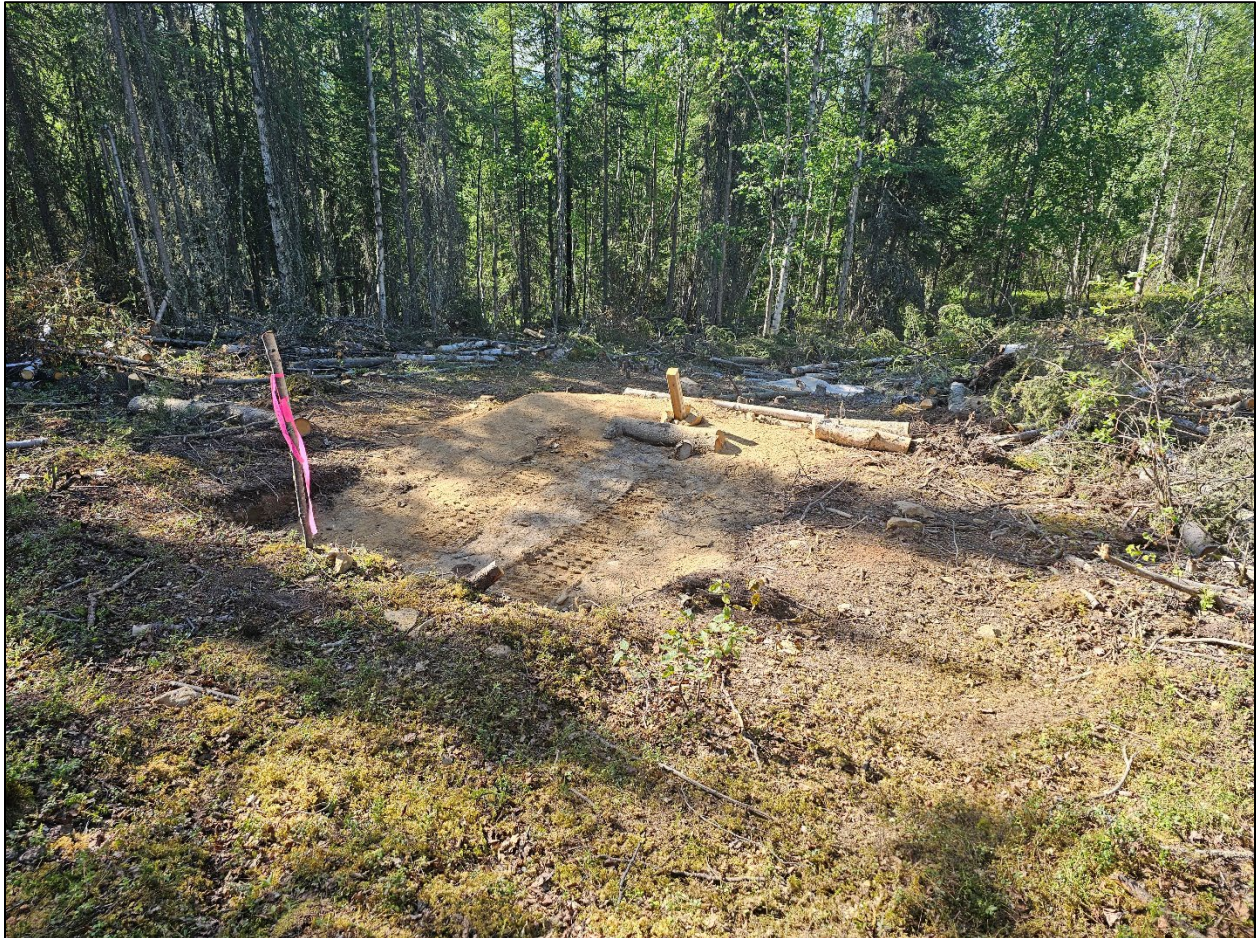
Photo 4. RAB pad requiring slight ground manipulation.
