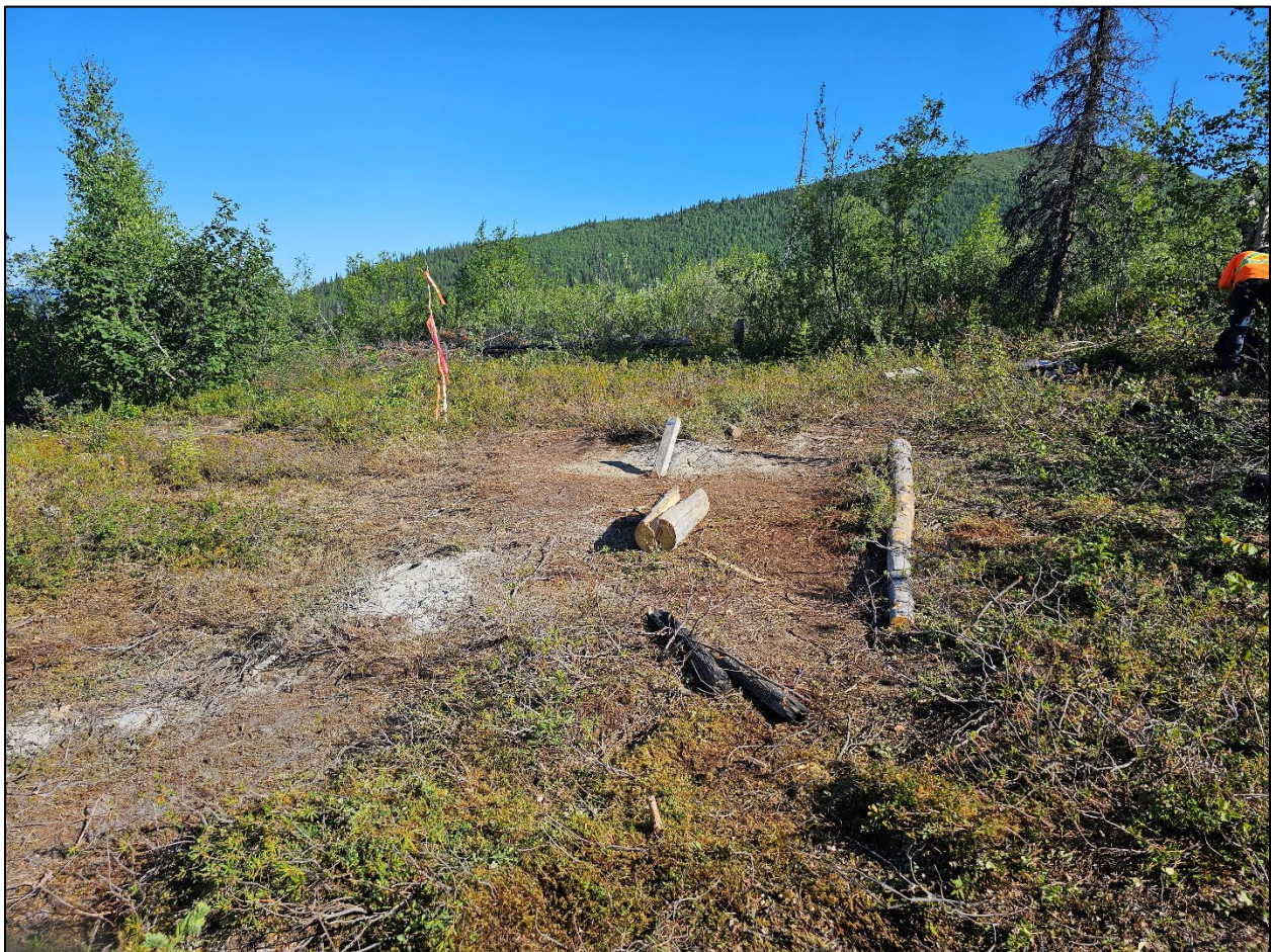
Photo 3. Typical RAB pad not requiring any ground manipulation or ground disturbance.
