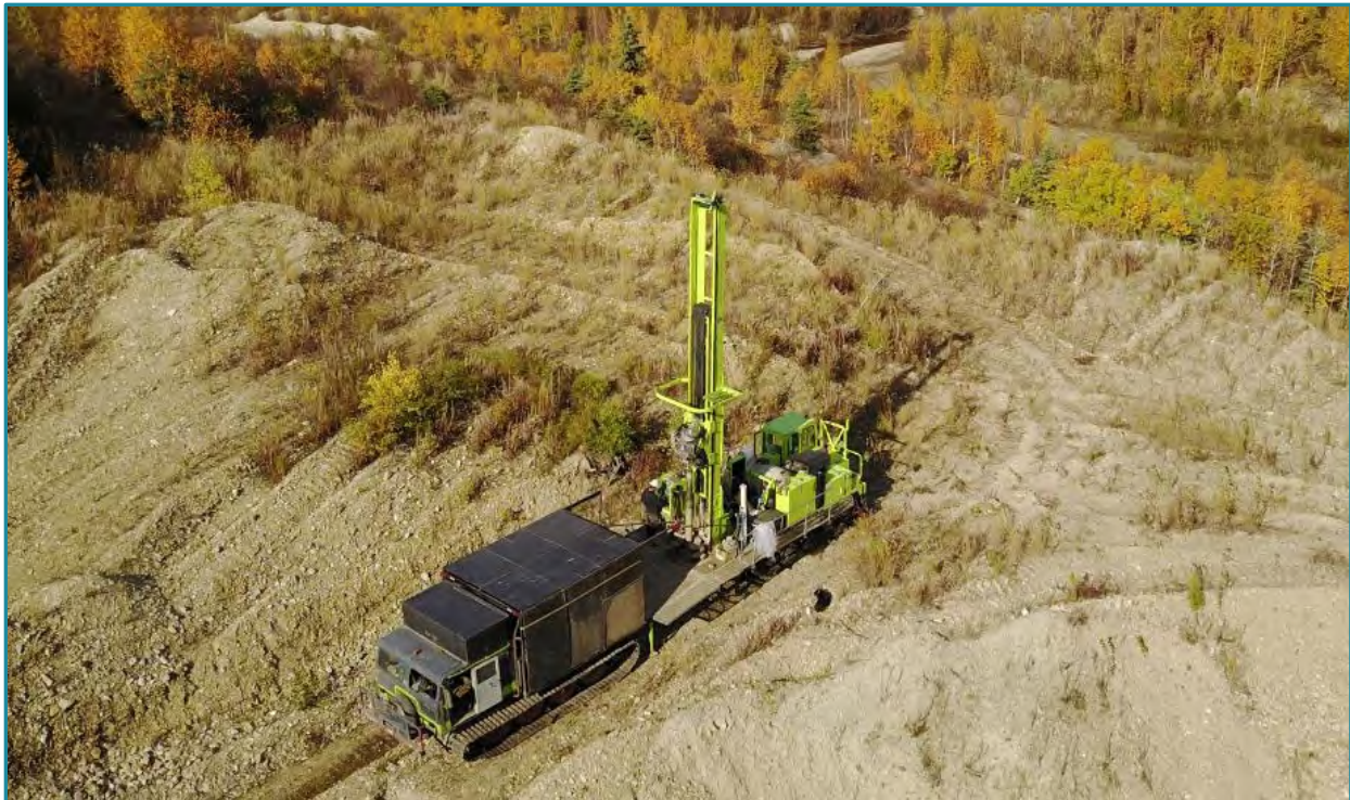
NSDC Terra Sonic Tsi 150c sonic drill rig and a Foremost TVS1000 support vehicle
