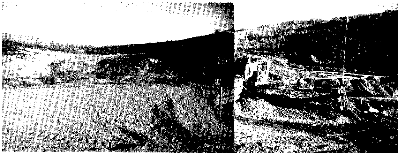
Panorama view of working area of pilot plant operation, Kenyon Creek, September 1976. View is looking east up the south fork of headwaters of Kenyon Creek; bulldozer at left centre and sluice box set up in foreground.
