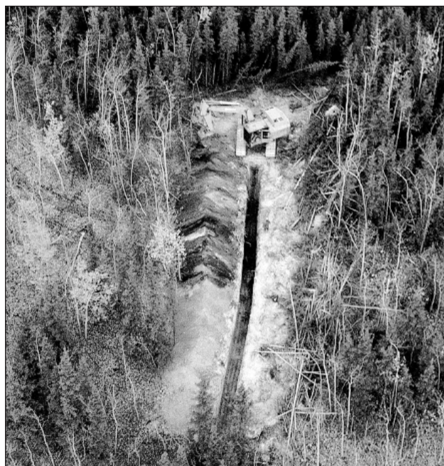
Figure 40. Coal can be seen in this trench excavated by Cash Resources on the Carmacks Coal Project. Cash also conducted a successful program aimed at expanding reserves at the Division Mountain Coal Project 70 kilometres to the south.
