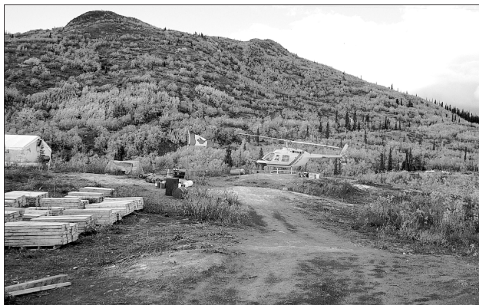
Figure 15. The Ice deposit of Expatriate Resources lies underneath the hillside behind the helicopter. Over 100 drill holes at 25- and 50-metre spacings have intersected the deposit in the area of this photo.
