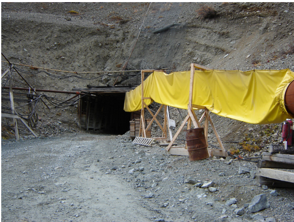
Figure 15. Skukum Creek property adit.
