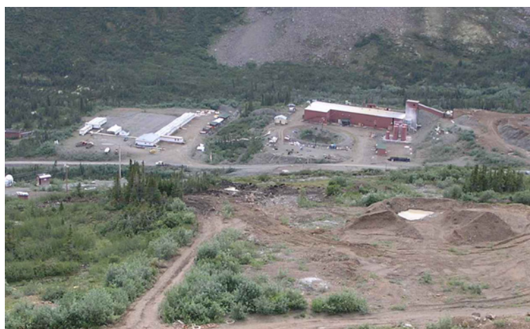
Figure 8. Ketza property, camp and existing mill.
