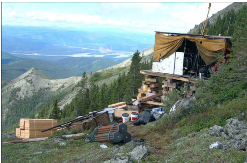
Figure 31. Drilling at Shell Creek.
