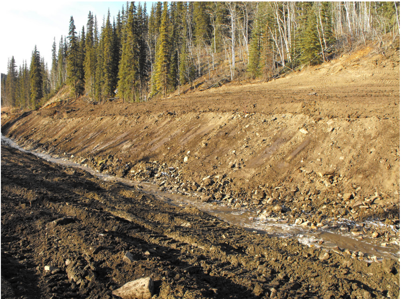
Figure 4. Re-sloped and contoured overburden piles along the creek allow for safe passage of migrating wildlife.
