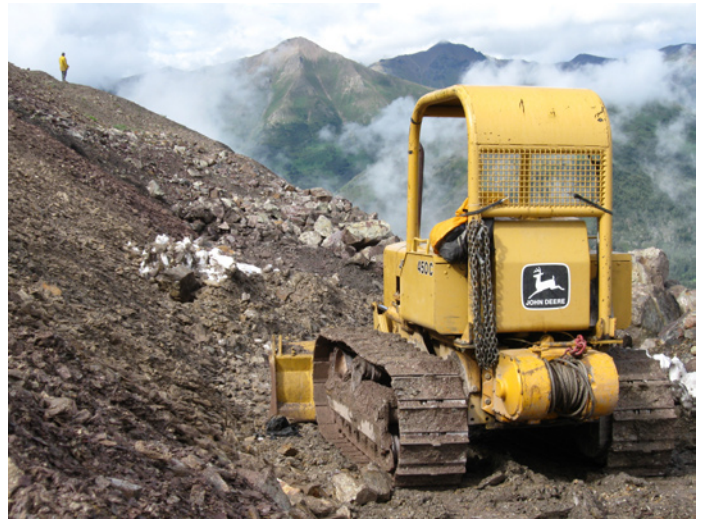
Figure 12. Trail building at the Plata property. Photo provided by Rockhaven Resources.
