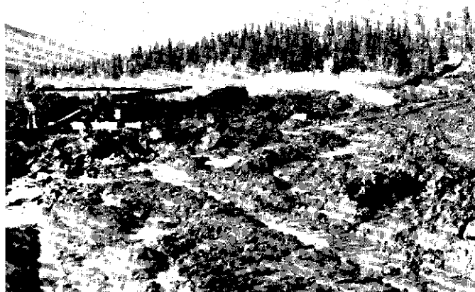
Hydraulicking to remove black muck from the D. Gritzka property along Sulphur Creek during 1982. A bulldozer was also used for stripping.
