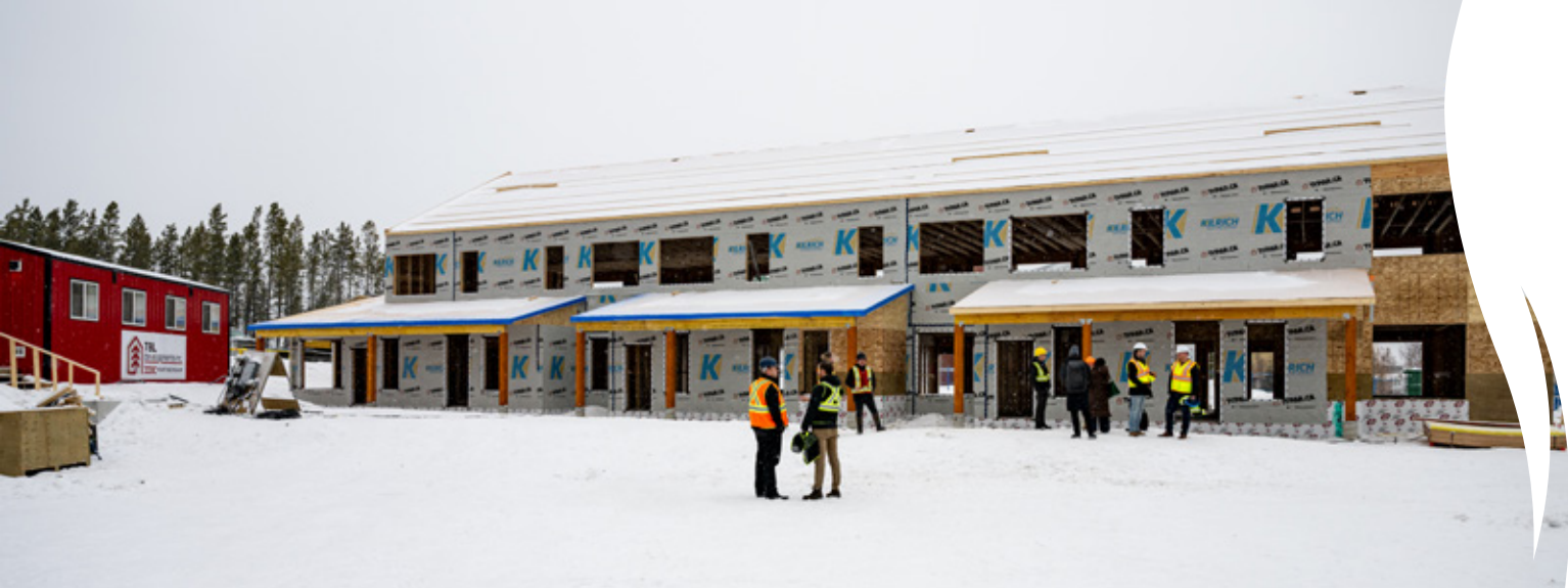
Winter Crossing construction. Canada Mortgage and Housing Corporation / Mark Kelly Photography
