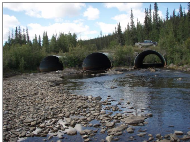
Figure 2.26: Culverts at the Davies Creek crossing (Photo: A. von Finster, DFO)
