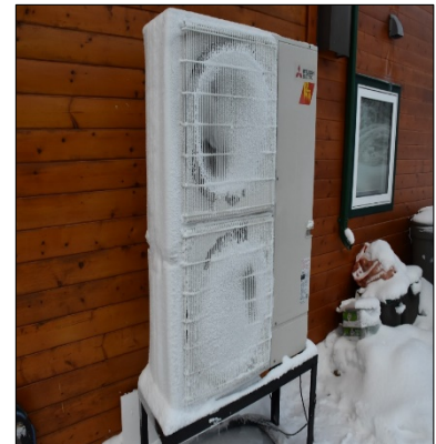
Figure 5: Overly iced-up Mitsubishi outdoor unit (42,000 BTU/hr).
