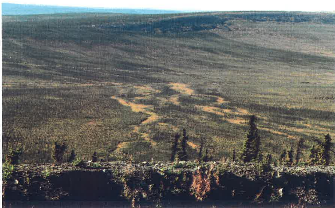
Photo D: Edge of sewage pit overlooking drainage to the Eagle River
