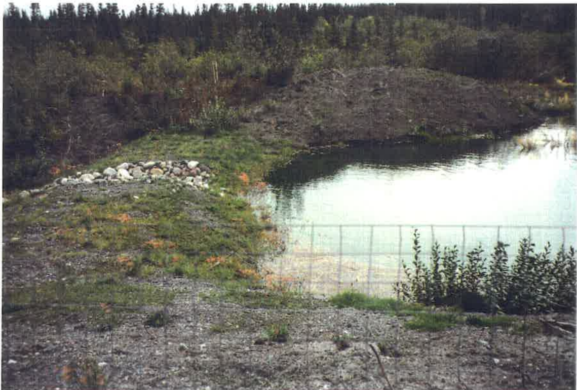
Photo H: Destruction Bay Sewage Lagoon - Level in Second Containment Pond
