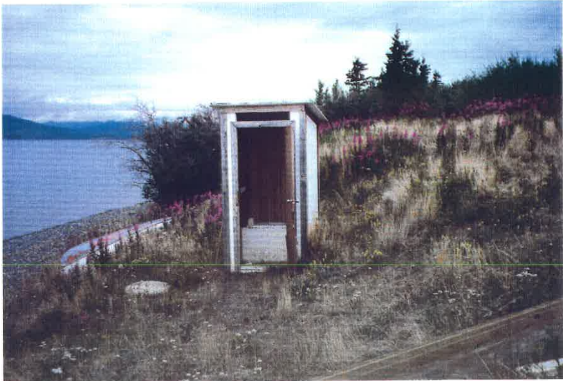
Photo Q: Burwash Landing - Pit Privy Above and Adjacent to Infiltration Well
