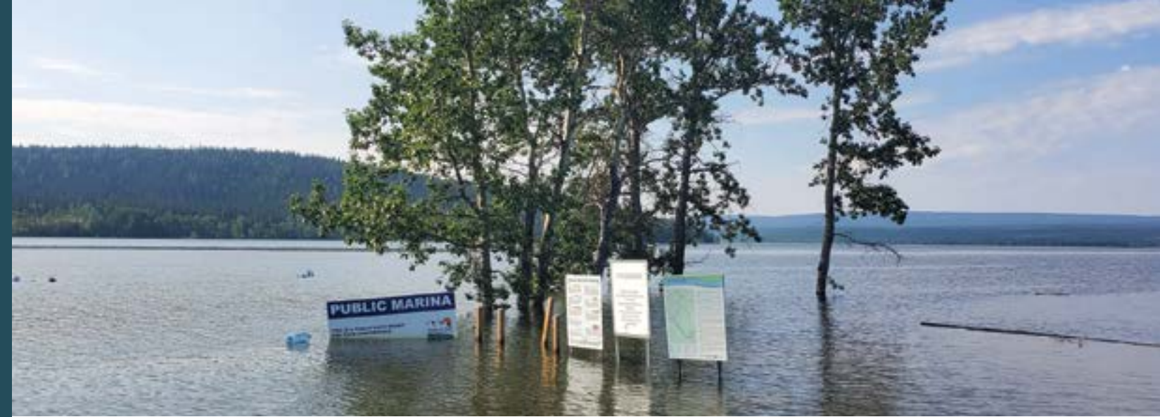
Teslin Marina signs during the 2022 flooding (Anthony Bier, 2022).
