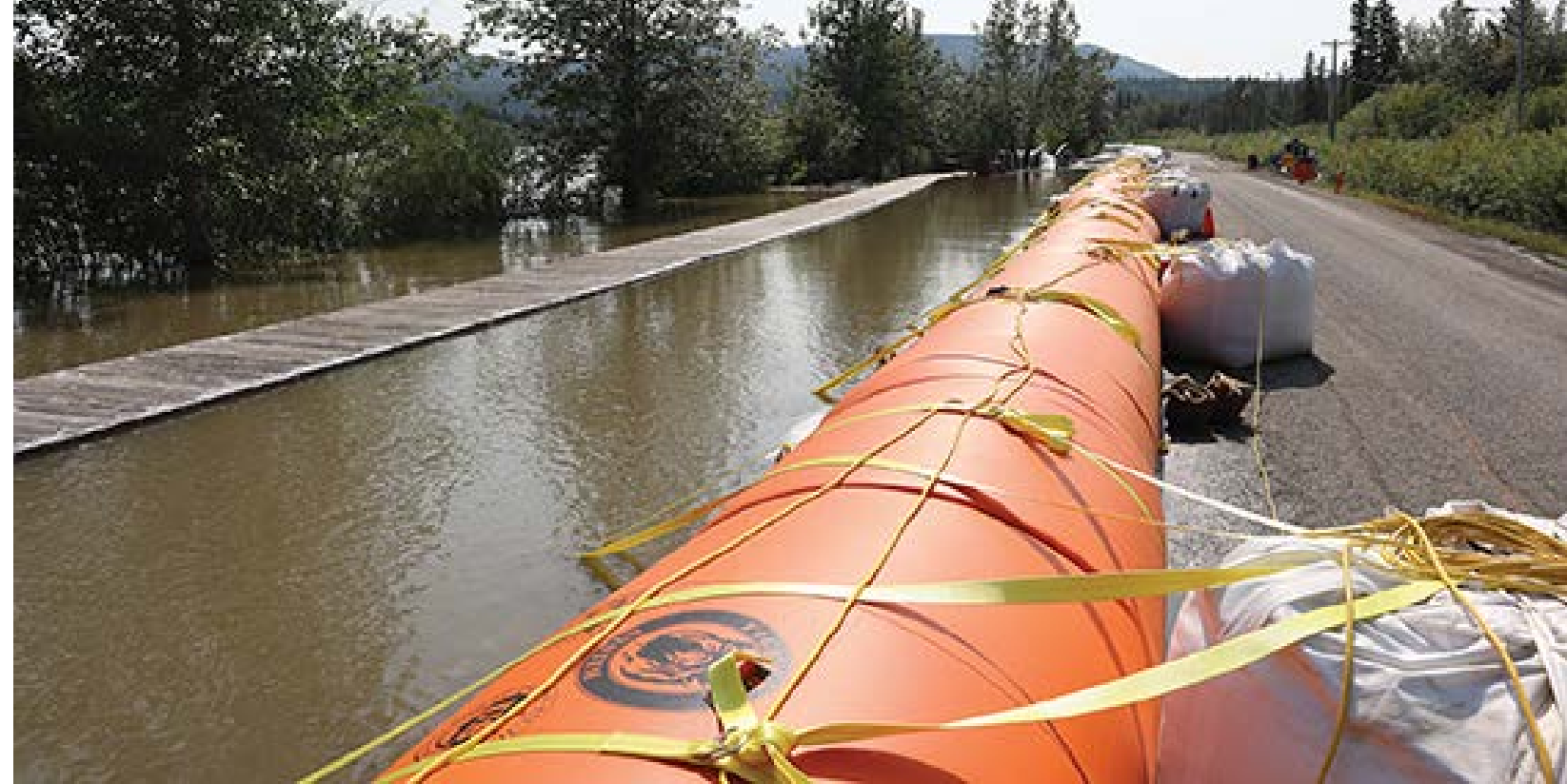
A Tiger Dam 3 set up on River Drive in Carmacks, Yukon (Anthony Bier, 2022)
