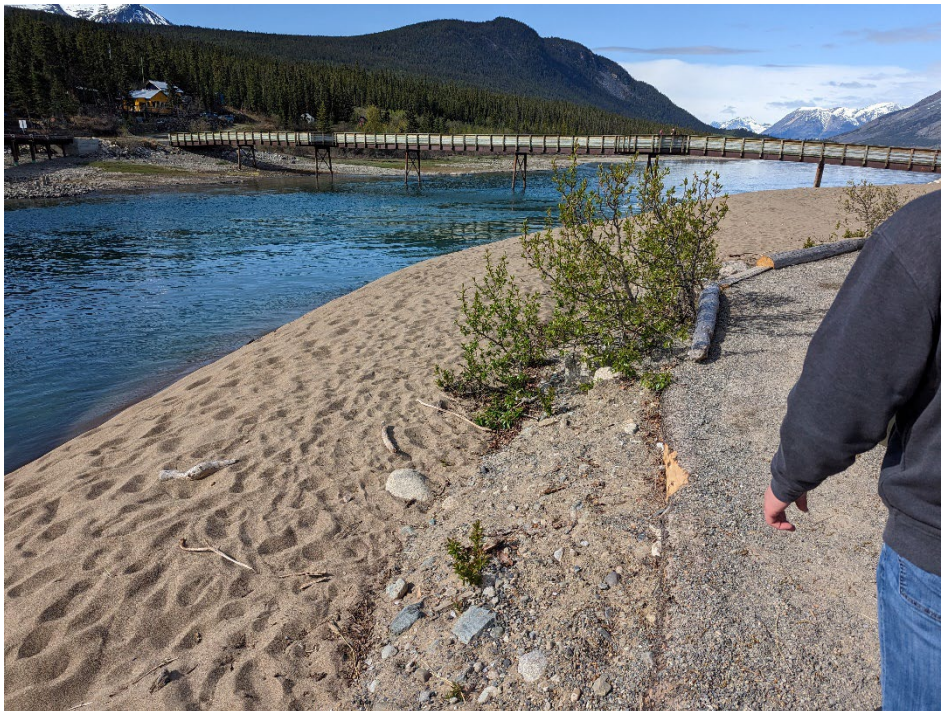
Photo 2: Pedestrian Bridge in Carcross
