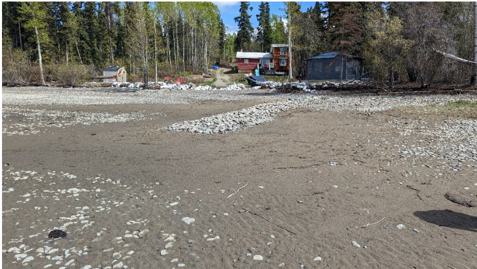
Photo 10: Temporary Flood Protection along Marsh Lake near Judas Creek
