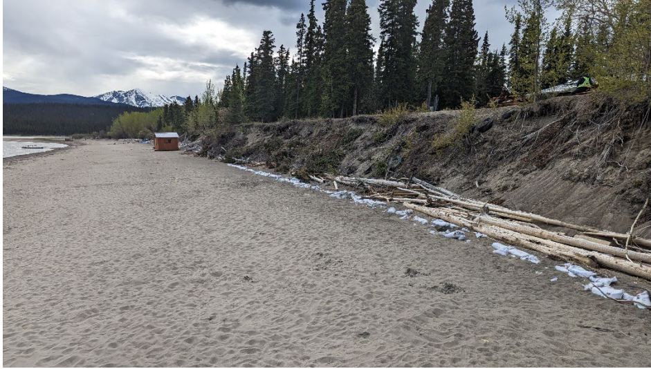
Photo 13: Temporary Erosion Protection on Marsh Lake Shoreline near Swan Haven
