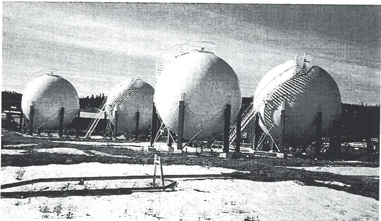
Figure 10. Spherical tanks at the petroleum depot, 31 March 1999. Midnight Arts photo
