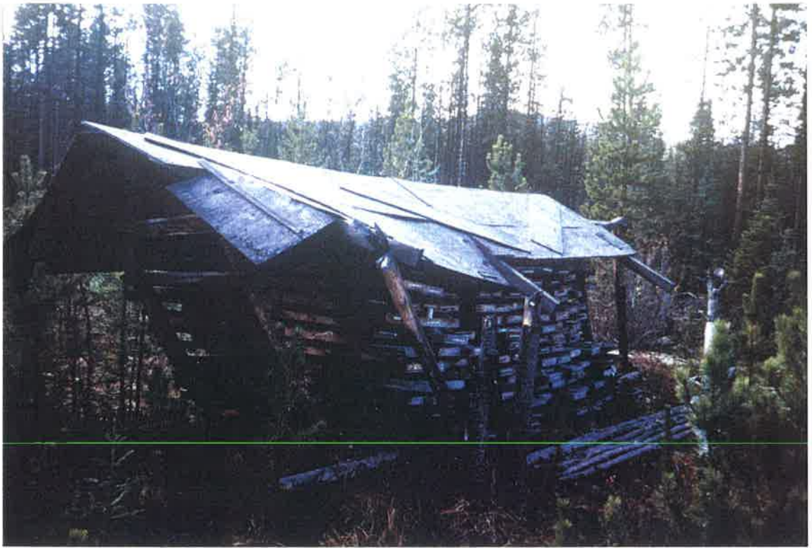
Photo 3: Site 1 - before reclamation
