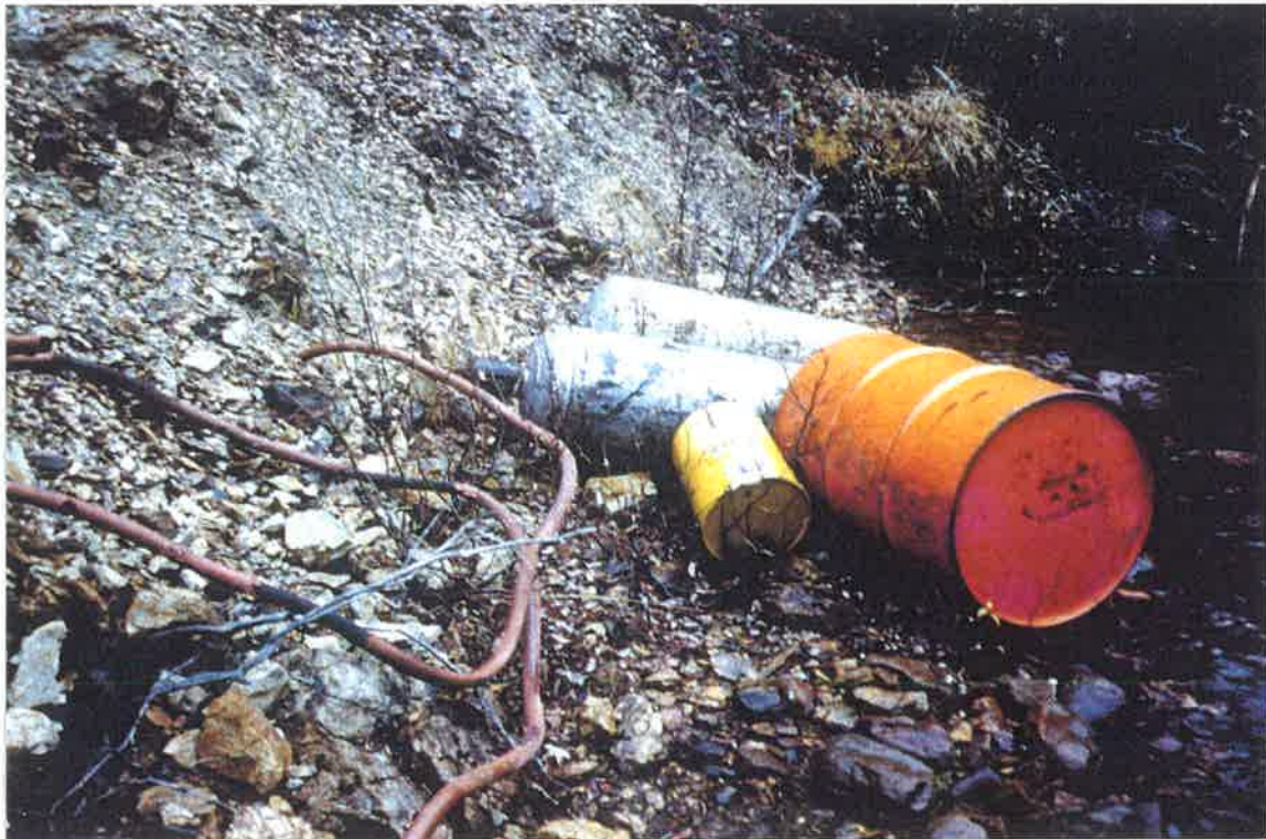
Photo 7: Site 2 prior to clean-up
