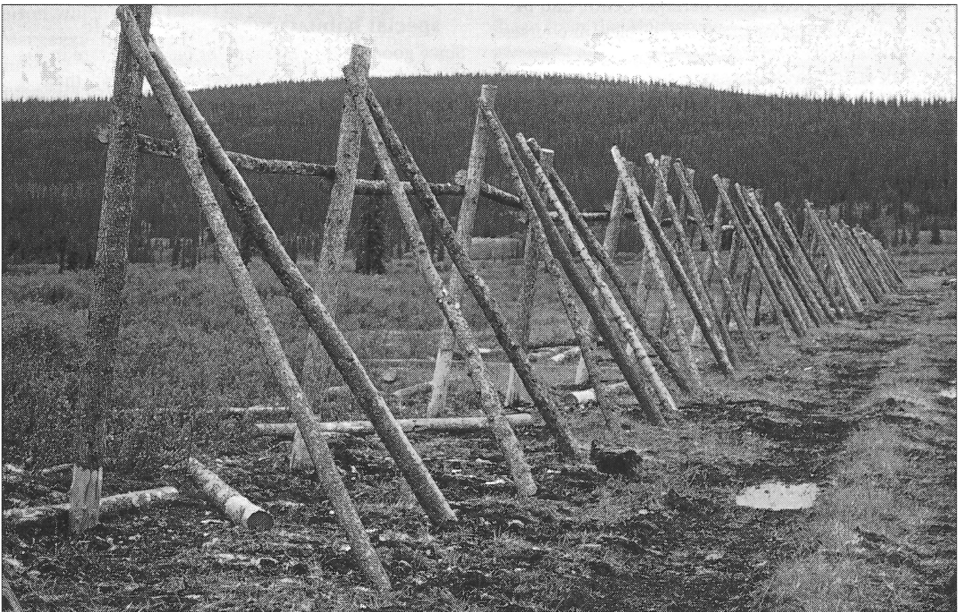
Enclosure fence construction in permafrost areas
