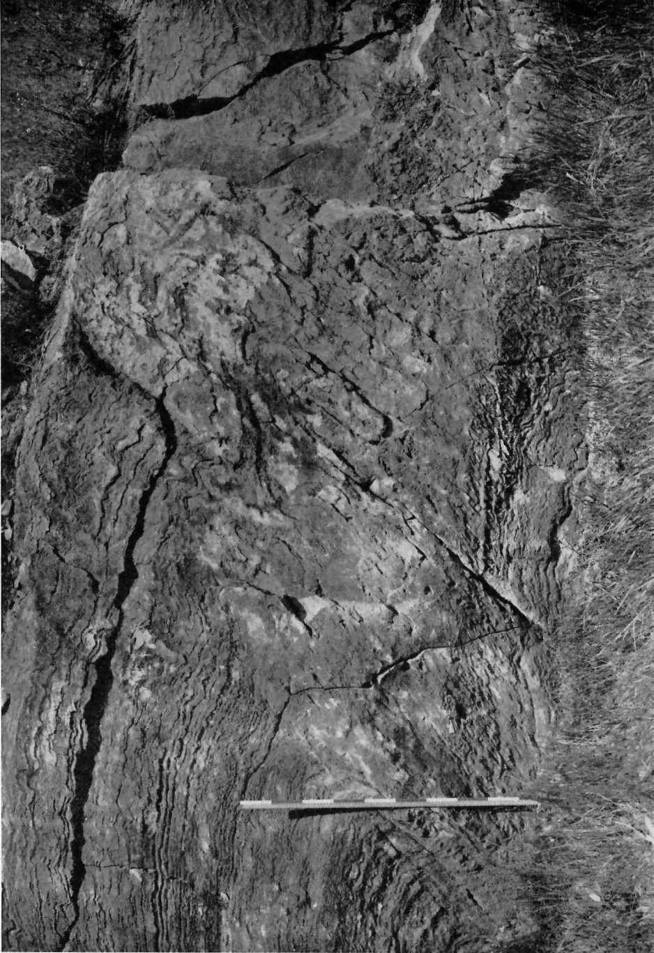
FIGURE 9. Elliptical structures grading into practically unfolded beds at left. Vertical section exposed in roadcut on Ontario highway 62 at L'Amable. The axes of the folds are nearly perpendicular to the face of the cut. Metre stick gives scale.
