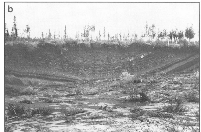
Figure 29. a) Retrogressive thaw-flow slide, southern Grand View hills, Travaillant Lake map area. In June 1950, the slide comprised a small area near the lakeshore; by 1973 when this picture was taken, it had retrogressed and developed three distinct embayments; note steep backwalls of active embayments and gently sloping floor. (ISPG 320-10); b) Backwall of embayment at upper right in Figure 29a; clay with reticulate network of ice overlies layered ice with intercalated layers of silty ice containing up to 40% silt. (ISPG 320-6)
