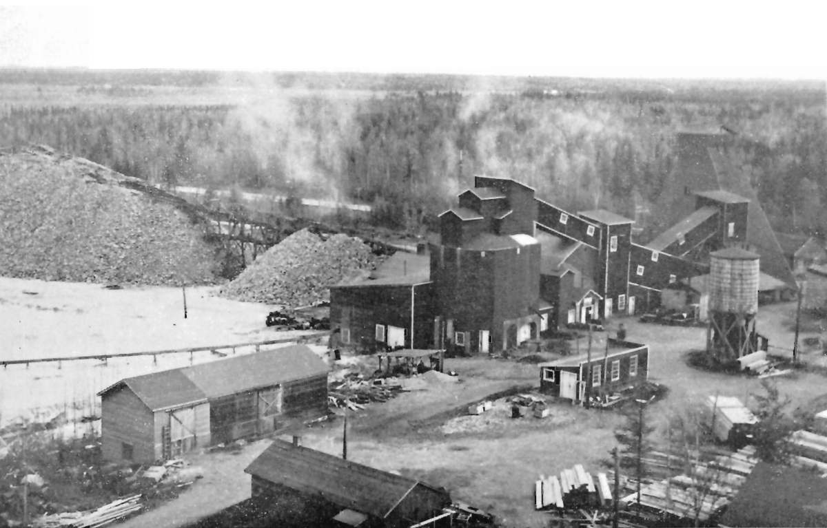
Plate 1. Headframe, concentrator and waste dump at the Lacorne mine of Molybdenite Corporation of Canada, Limited (June 1958).
