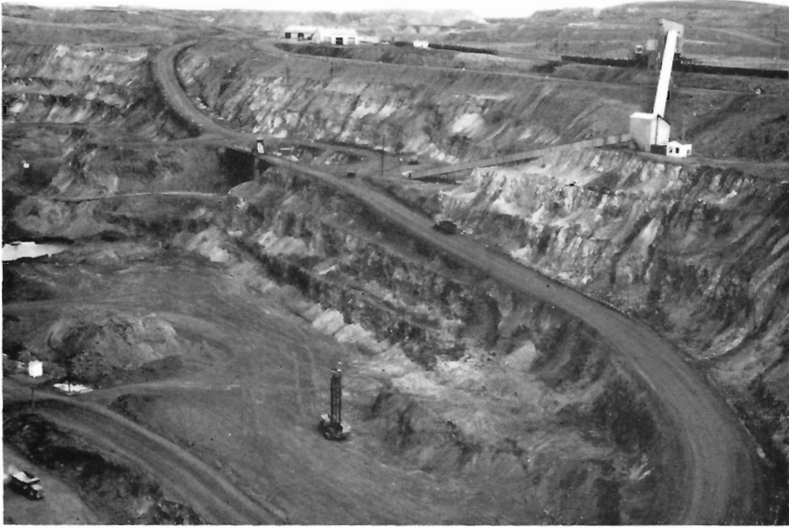
A. Ore conveyor system and loading station, Gagnon A mine, Quebec, 1962.
