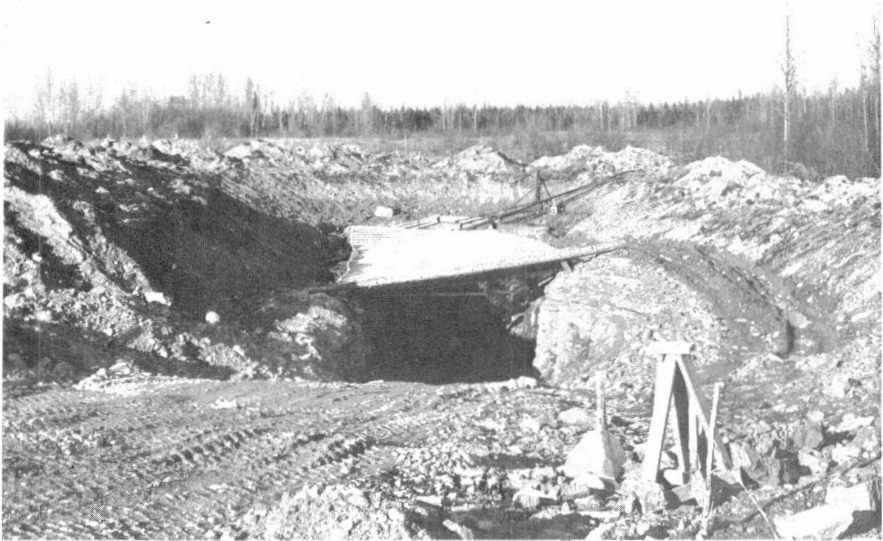
Figure 3B. St-Honoré Niobium Property Camp – portal to the 20 per cent decline to develop orebodies 1 and 2.
