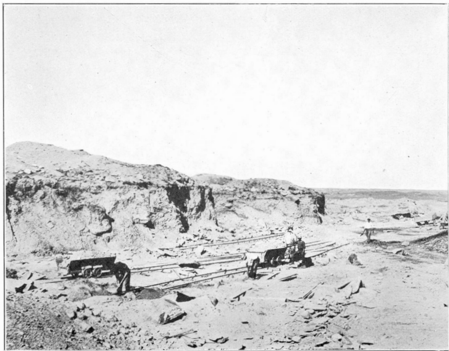
Surface deposit of glacial clay, used for stiff-mud bricks, Estevan Brick and Coal Co.
