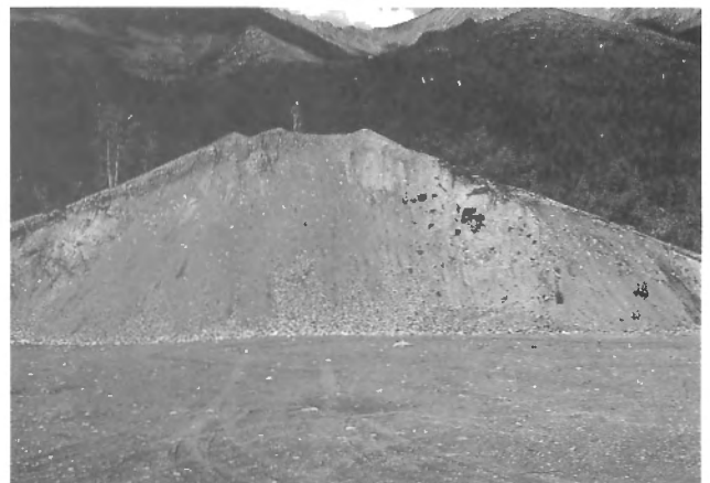
Figure 20. Borrow pit face across a crevasse filling on the west side of Nahanni Range Road, northeast part of the Dolly Varden Creek map area (Map 1674A). Top of feature flattened by bulldozer. GSC-203603-Q
