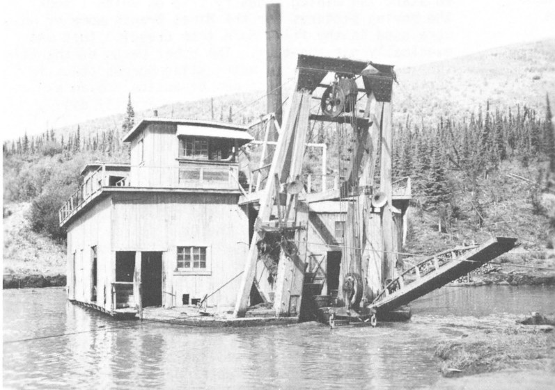
The wood-burning steam dredge at Sixtymile River in 1936 when it was being worked by E. Holbrooke. (81612).
