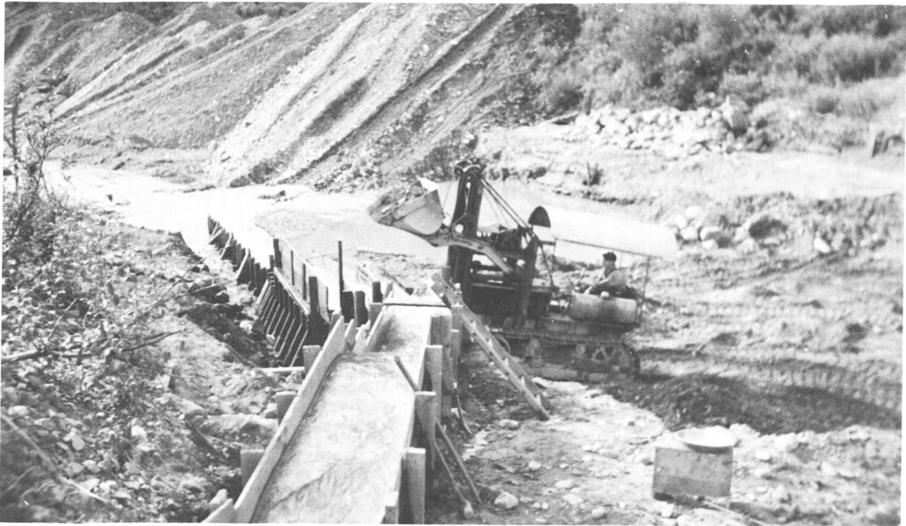
Placer mining at Haggart Creek. Gold-bearing gravel is being dumped into silver box. (88544)
