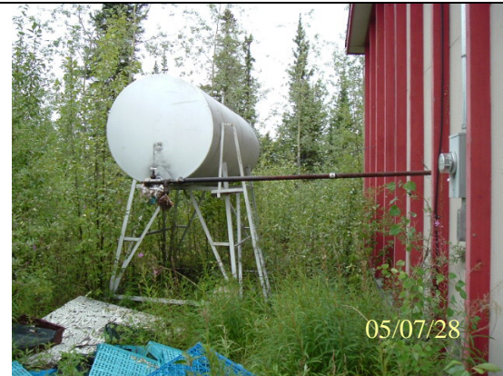
Photo 0575: 3102 Above ground fuel storage tank behind firehall
