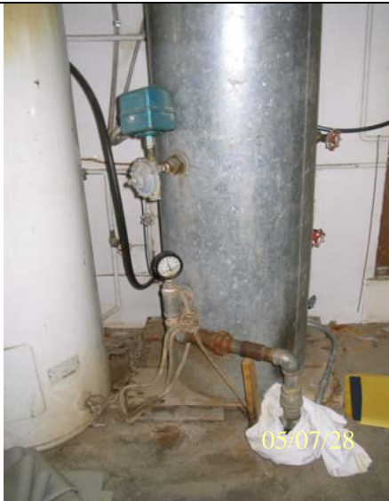
Photo 0104: 3102 Wellhead (bottom), pressure tank (top). Note well casing is covered with a piece of cloth
