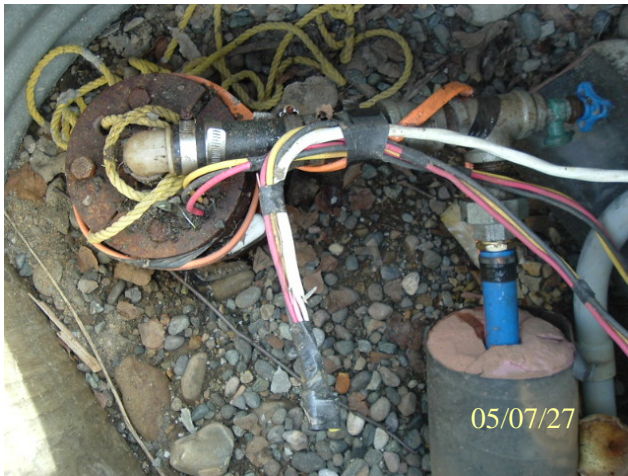
Photo 0561: 3121 Wellhead in pit
