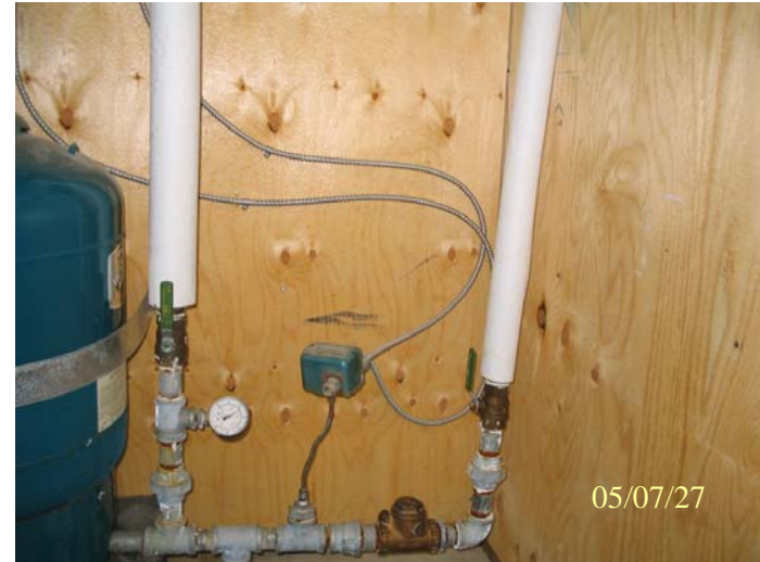
Photo 0099: 3121 Point of entry and pressure tank
