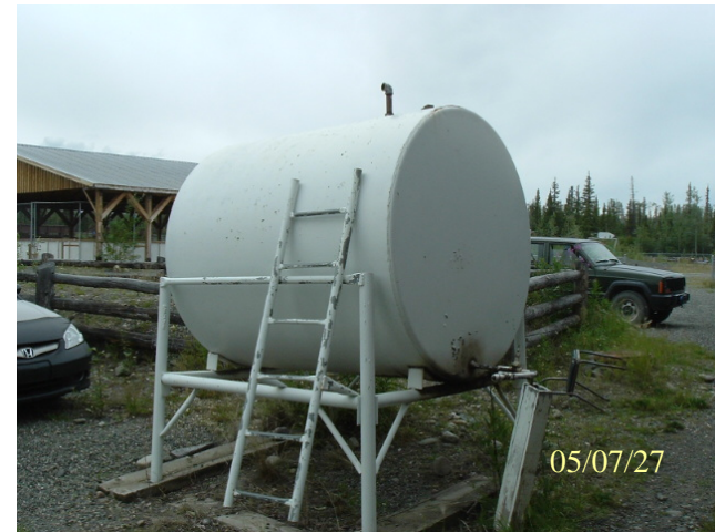
Photo 0539: 3122 Above ground fuel storage tank
