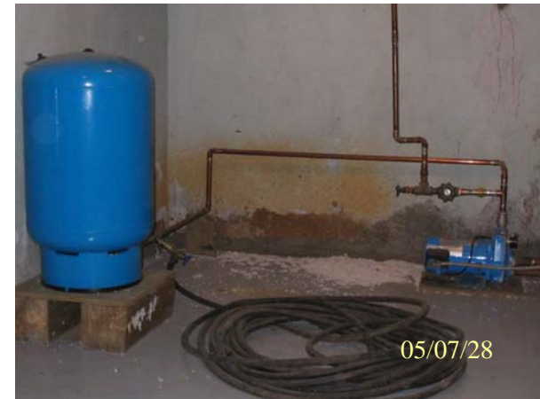
Photo 0114: 3201 Pressure tank (left), and jet pump (right)
