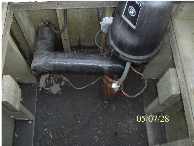
Photo 0615: 3171 Wellhead in pit, pellet chlorinator
