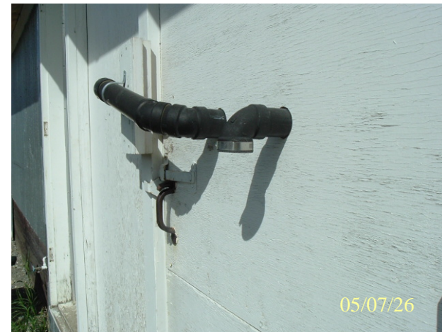
Photo 0511: 3443 Warehouse ABS fill pipe
