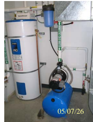
Photo 0067: 3443 Jet pump and pressure tank (centre), water heater (left)
