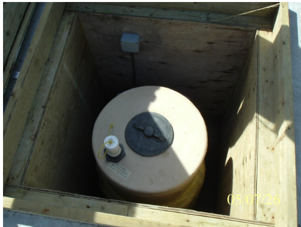
Photo 0505: 3443 Underground water storage tank
