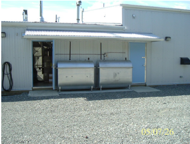
Photo 0504: 3443 Above ground fuel storage tanks
