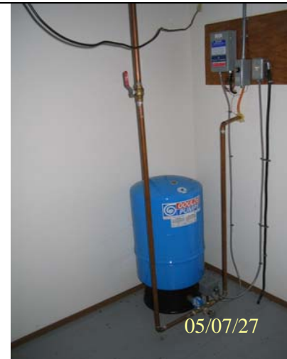
Photo 0094: M0134 pressure tank and pump controls
