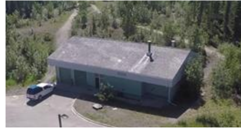
The biomass system will be installed in the boiler building at Elijah Smith Elementary School in Whitehorse, Yukon.
