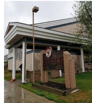
Watson Lake High School is heated with waste heat from the town's generators.
