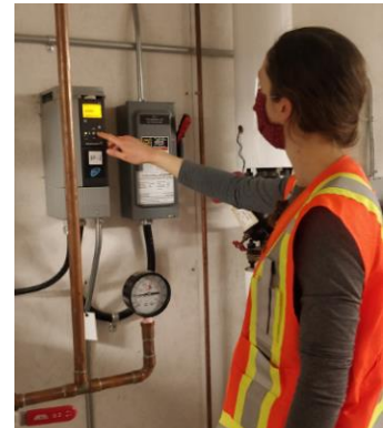
Loreena Dobson, our Energy Technical Specialist, inspects equipment at a building.
