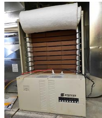
Electric Thermal Storage units convert electricity into stored heat.
