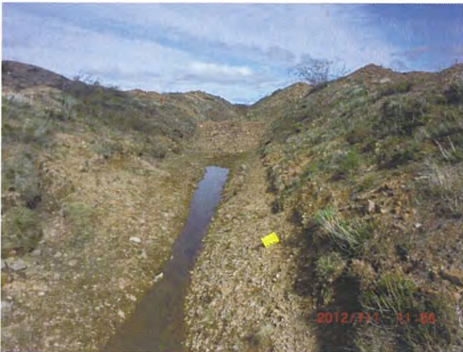
Existing Open Trench
