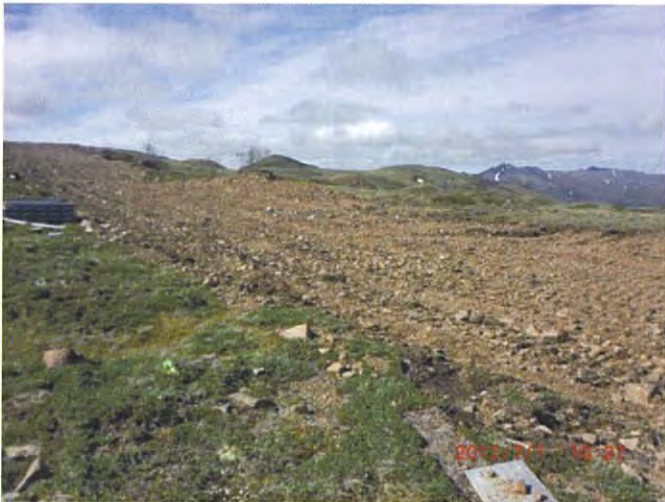
Reclaimed and re-contoured trench on Vic property
