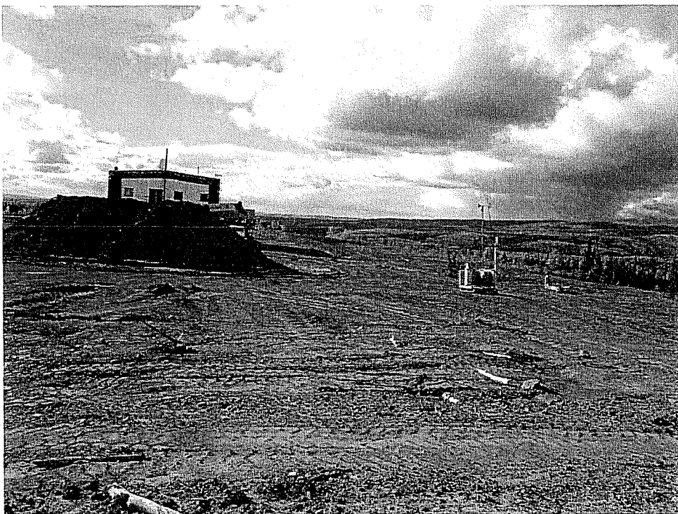
Plate 8. Main Fuel Storage Area - Site MF-S-#6.
