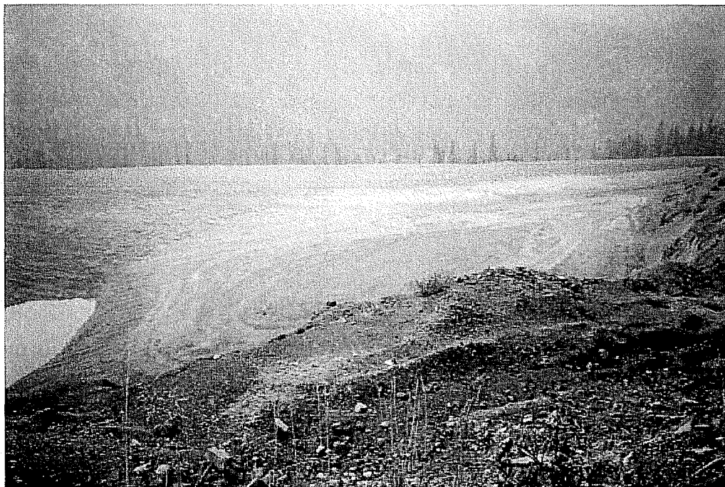
Kokanee: Looking at the backfilled pit area. August 17, 2005.
