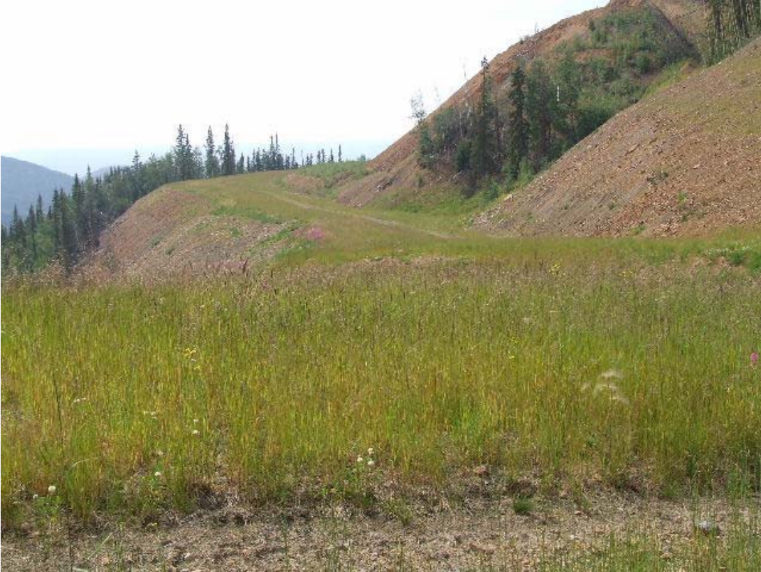
Haul Road just north of Canadian Zone. July 19, 2006
