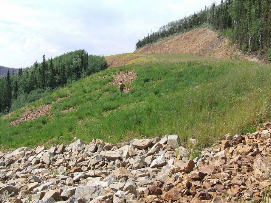
Flanks of Haul Road at one of the stream crossings. July 19, 2006.
