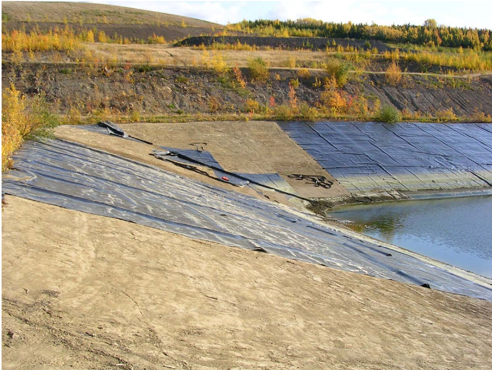
Liner removed from overflow pond
