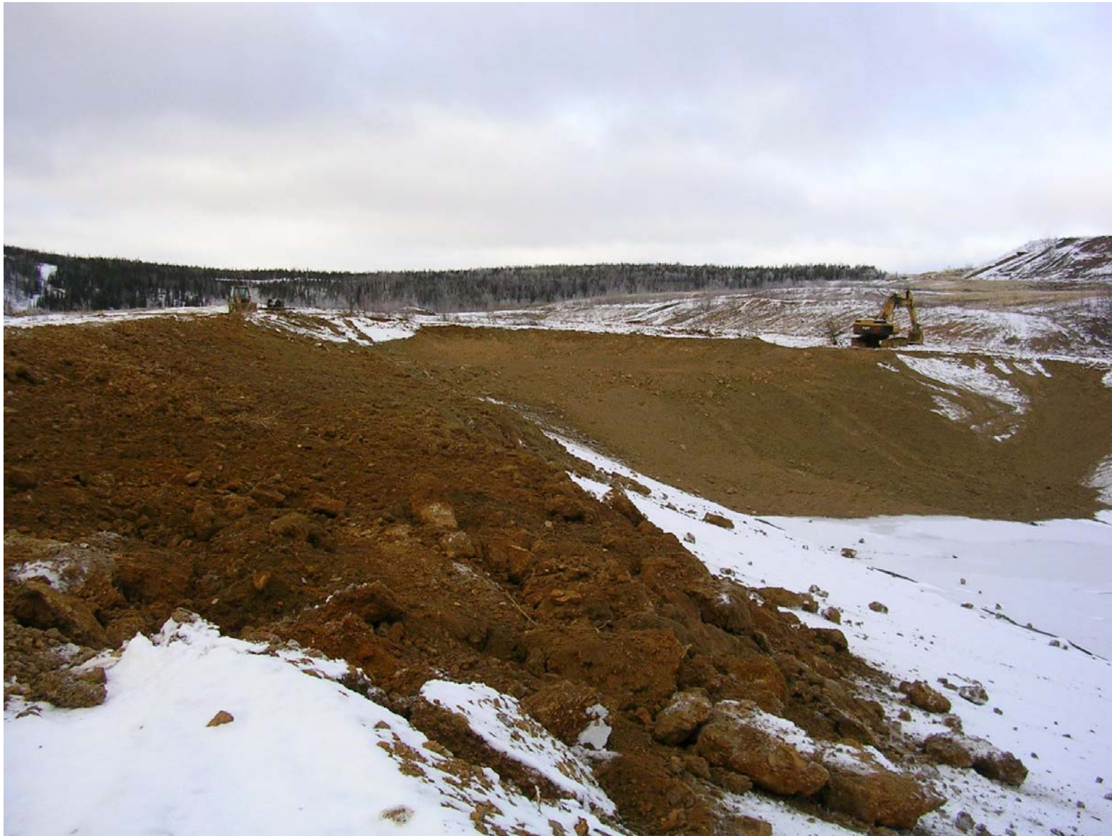
Final recontouring of overflow pond
