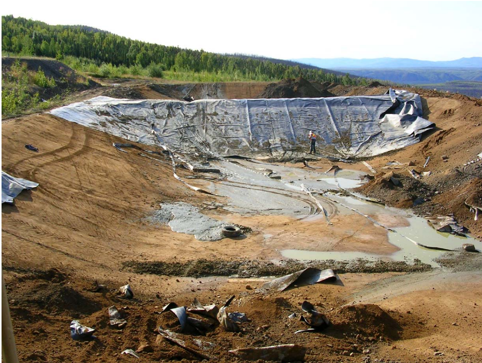
Removal of liner in water treatment ponds
