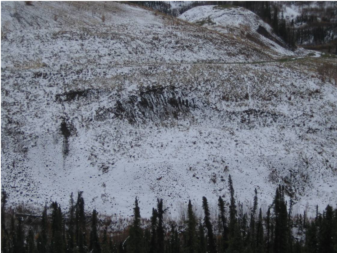
Photo 14: Taken from “Photo Hub #1”, view of the slope instability below the Lucky Dump haul road.
