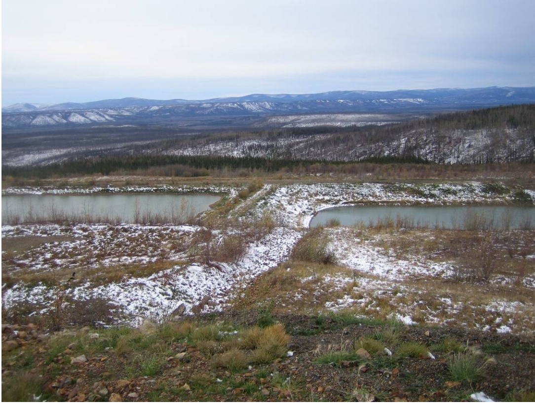
Photo 25: View of the rip-rap lined channel below the breach leading to the former Pregnant Pond.
