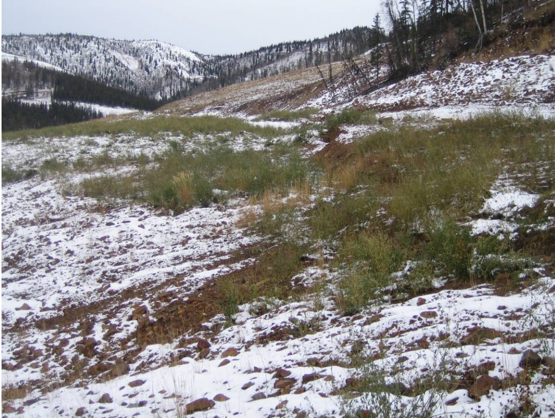
Photo 17: View of the scarp at the second failure location. The scarps are up to 1 m in height.
