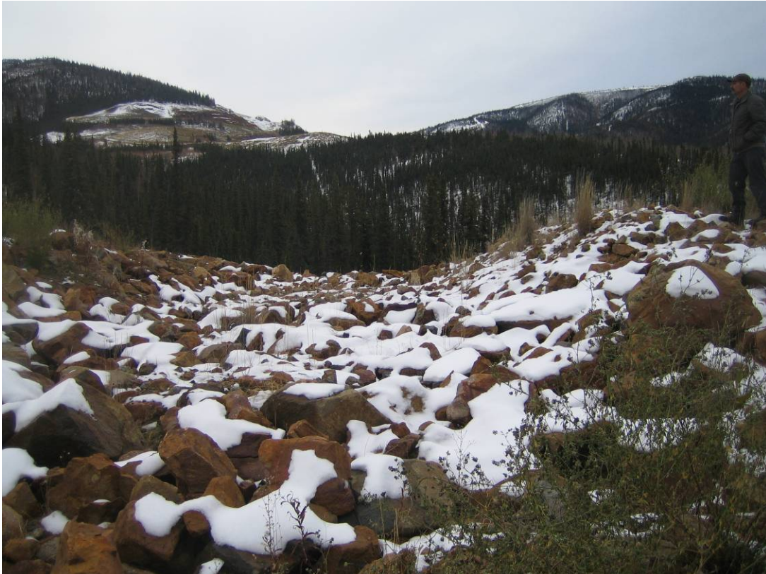
Photo 10: View of rip-rap placement at the Blue Pit outfall placed in 2009.
