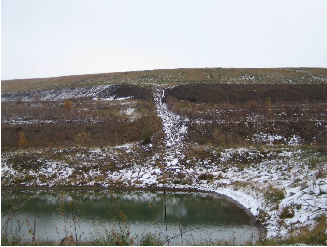
Photo 27: View of the heap leach breach leading into the former Pregnant Pond.
