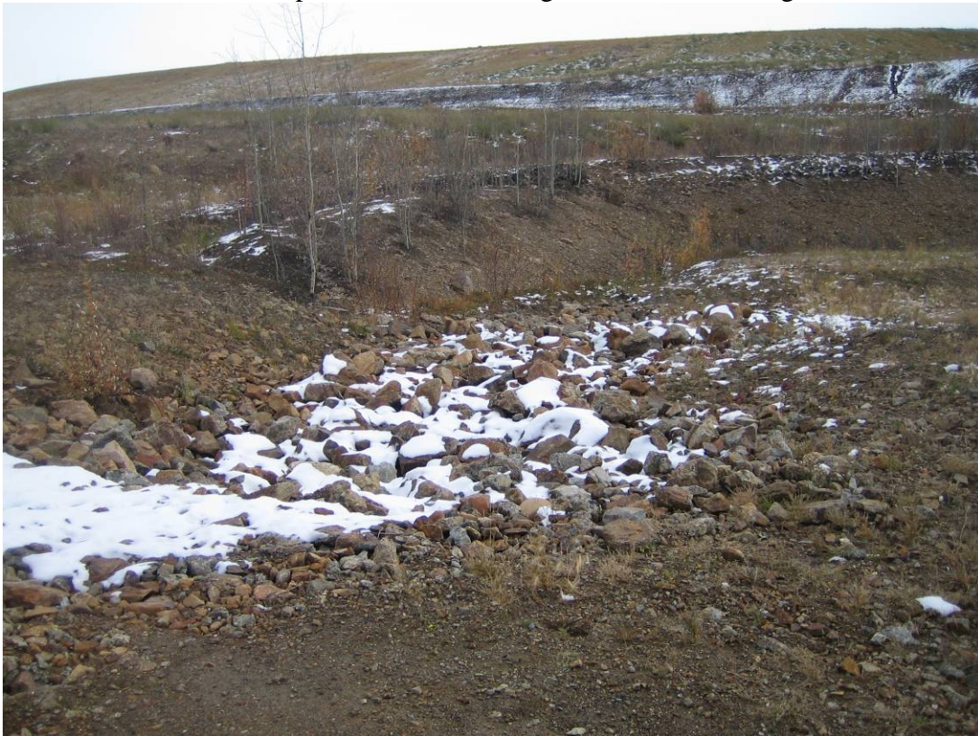
Photo 28: View of the overflow channel on the west side of the former Pregnant Pond to the south.
