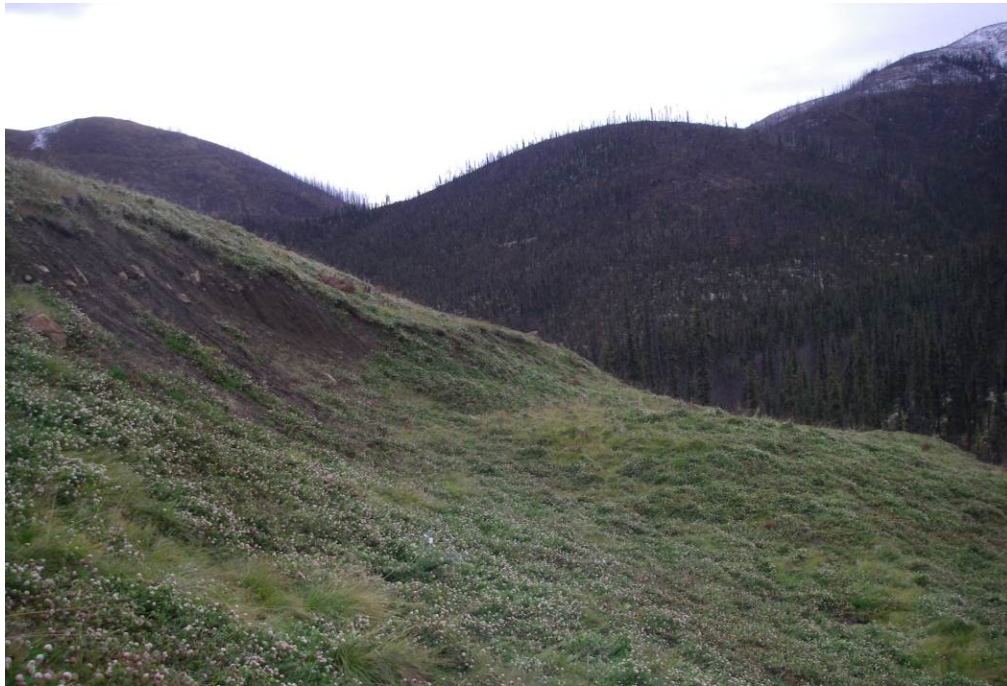
Photo 9: View of the slope instability below the Lucky Dump haul road taken from just east of the area.
