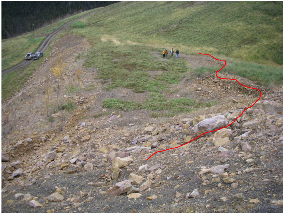
Photo 15: View looking towards the west. The Lucky Pit is located to the right of the photo, main access road to the left, and 2 nd failure (photo 10-12) further to the left. Approx. locations of scarps/cracks are noted in red. These features were not noted in the 2010 inspection, possibly due to snow cover.
