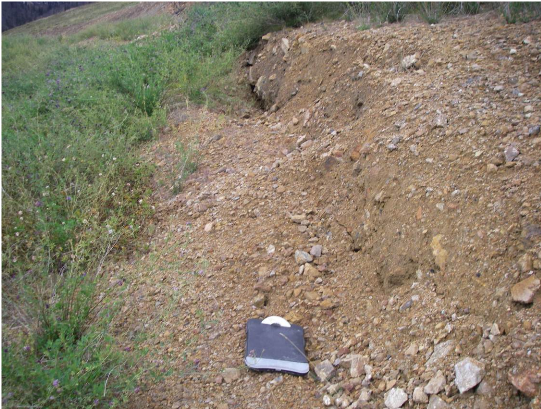
Photo 11: View of the scarp at the second failure location. The scarps are up to 1 m in height.
