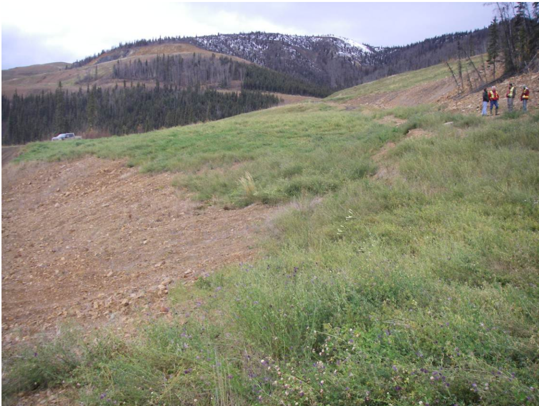
Photo 10: View of the second failure location by the Lucky Dump haul road above the Bohemian Access Trail, taken from "Photo Hub #4".
