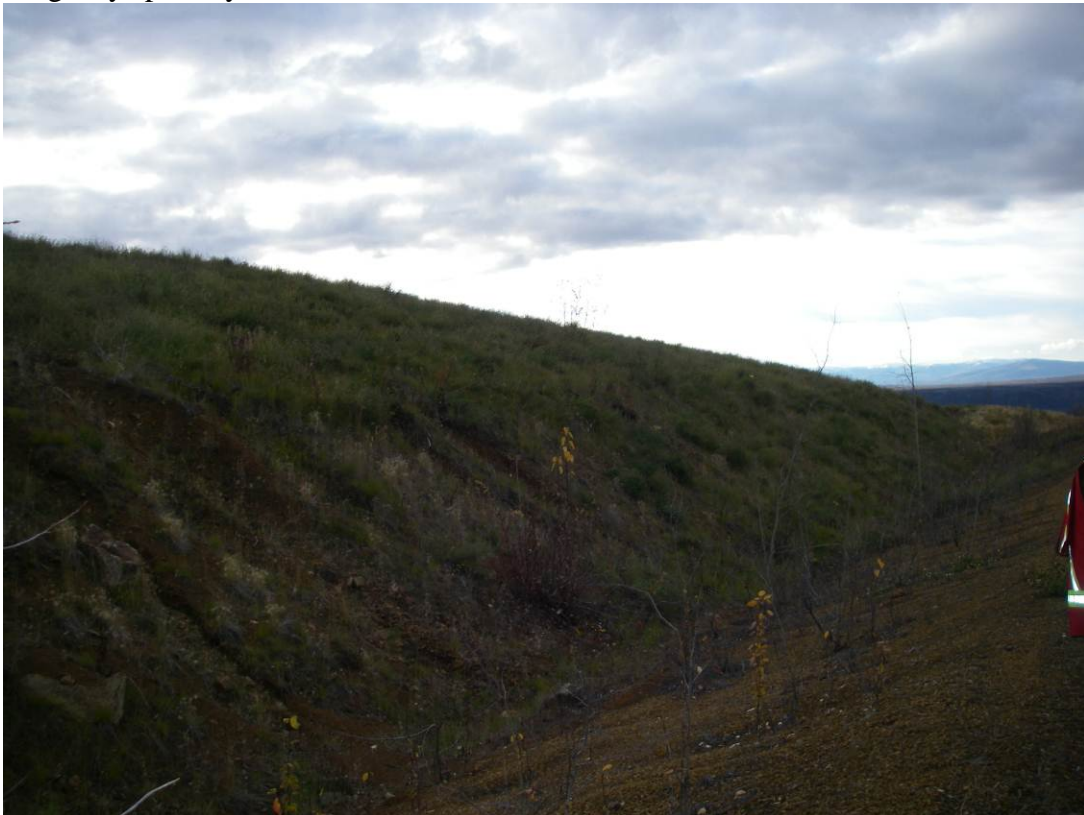
Photo 18: View of gullies at the base of the heap leach pad above the dyke near the breach (visible to the right of photo). Vegetative growth is occurring within the rills indicating the gullies are stabilizing.
