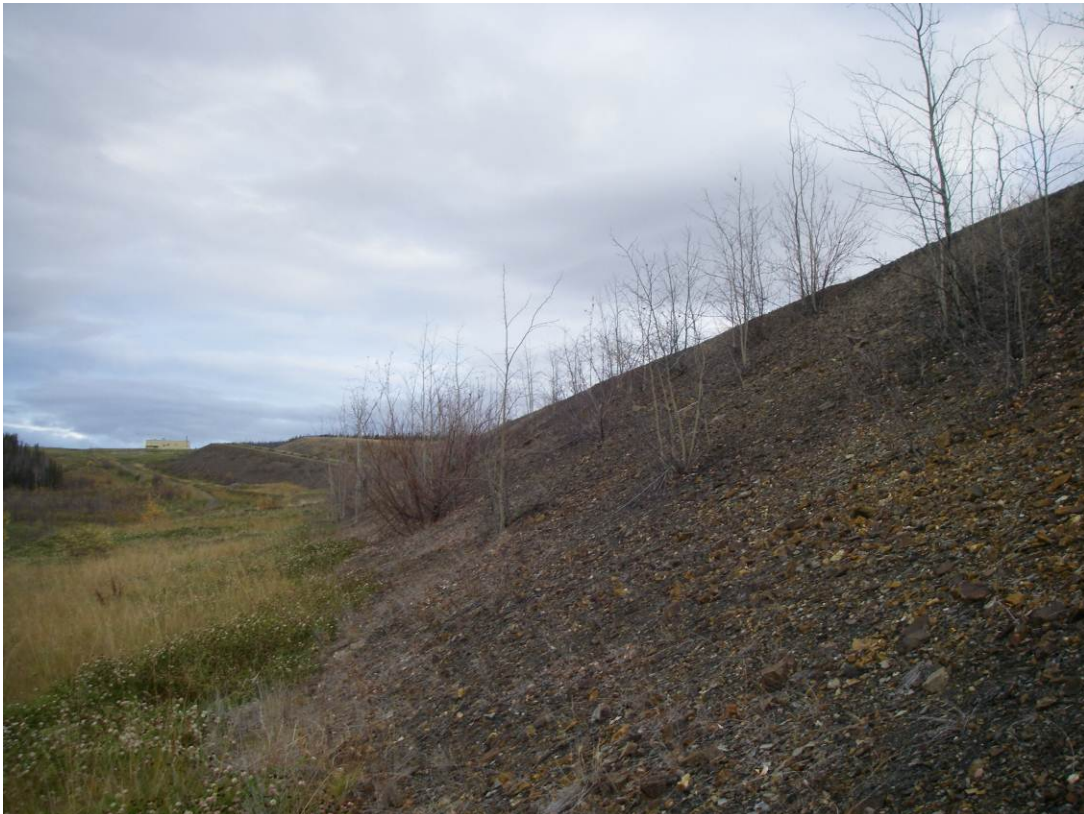
Photo 20: View of the heap leach containment dyke looking north.
