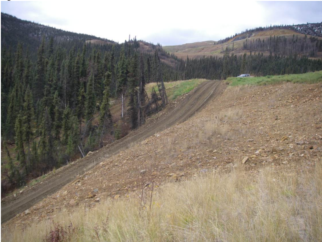
Photo 12: View of the slope above the Bohemian Access Trail.
