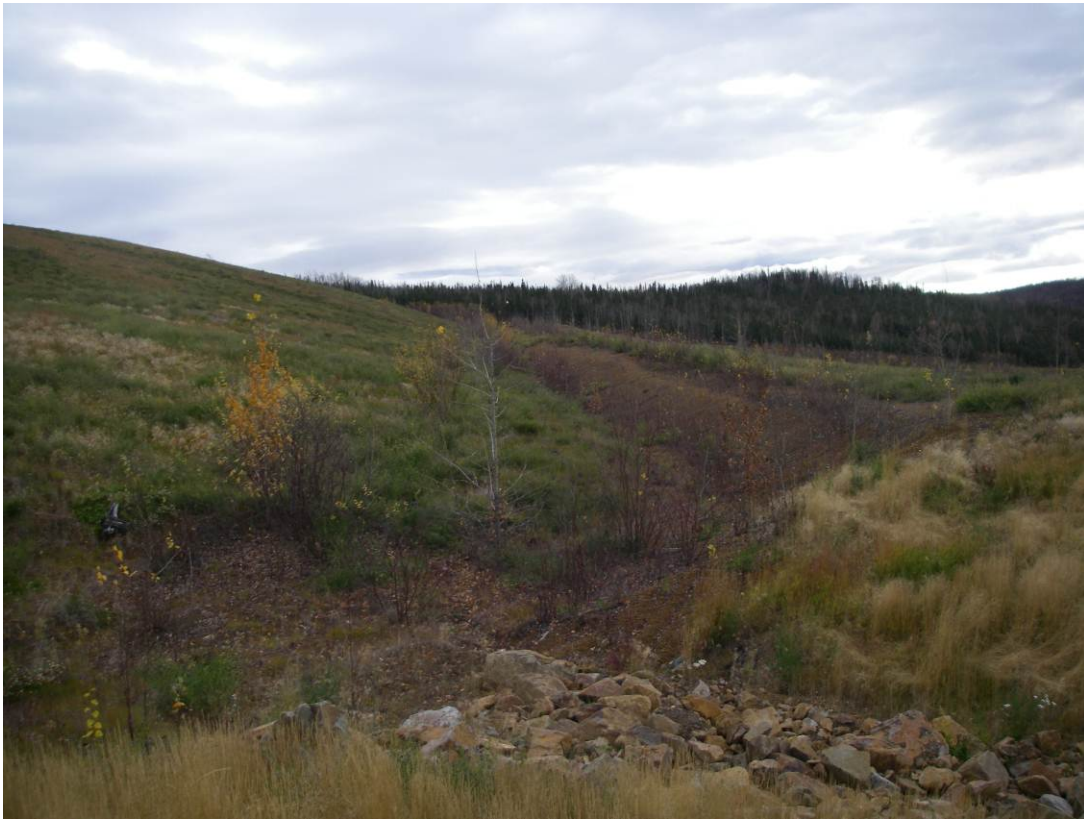
Photo 17: View of breach completed in 2009 of the heap leach pad dyke at the former emergency spillway location.
