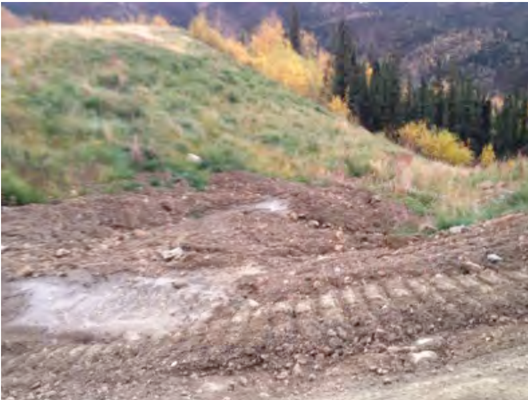
Plate 8: Haul Road Swale KP 3.2 - Repaired Washout
