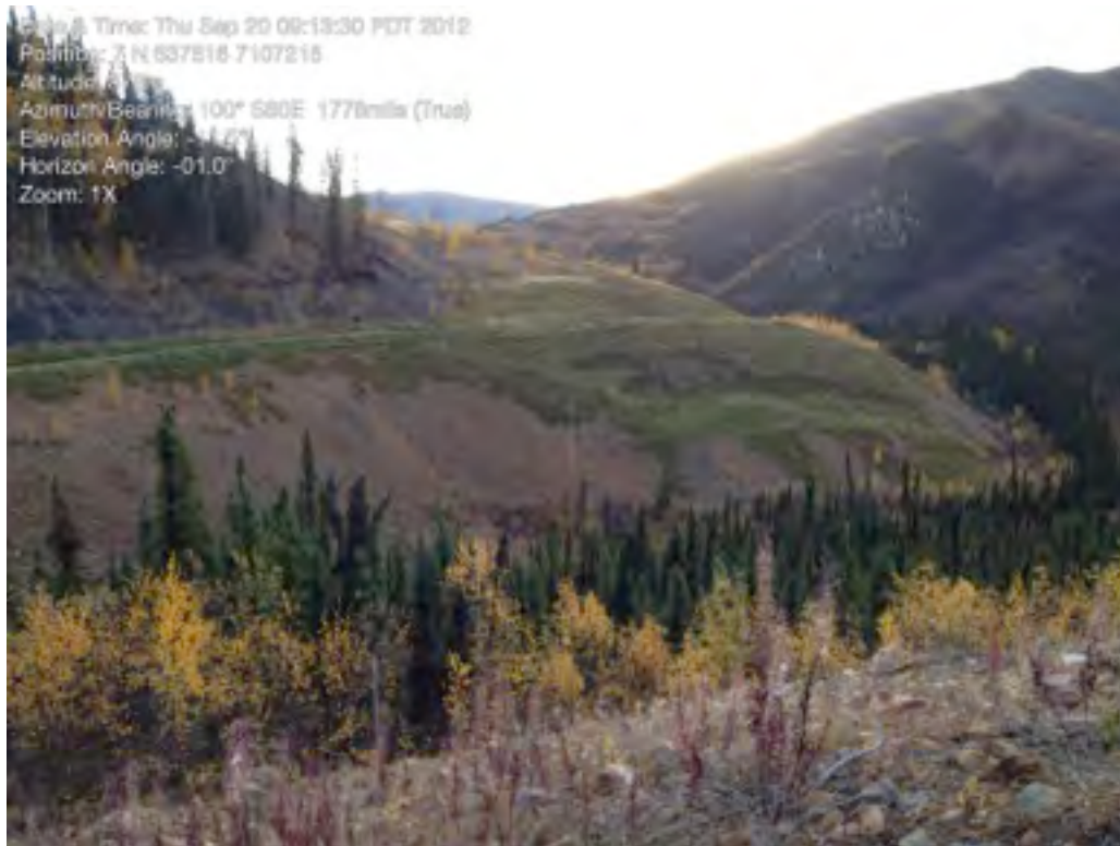
Plate 12: Road Embankment at Luck Haul Road
