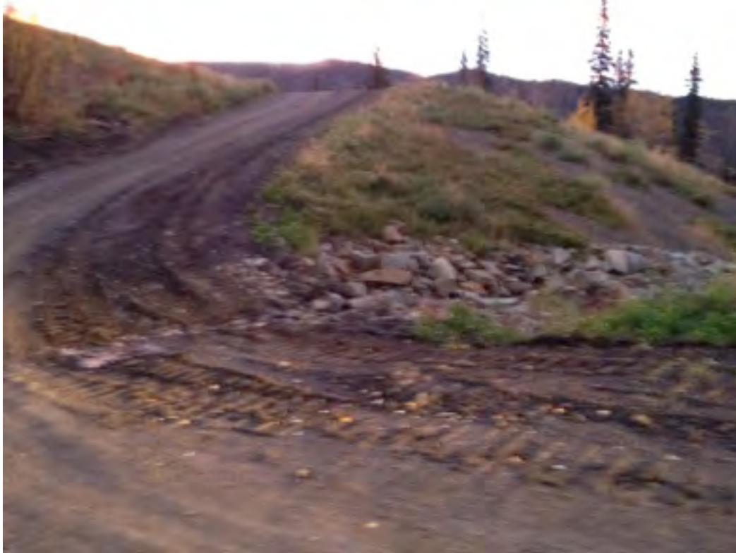
Plate 5: Haul Road Swale Discharge KP 1.5
