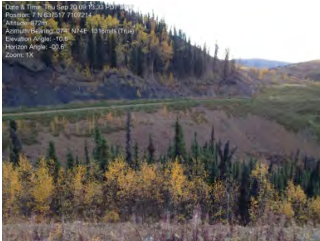
Plate 11: Road Embankment at Lucky Haul Road
