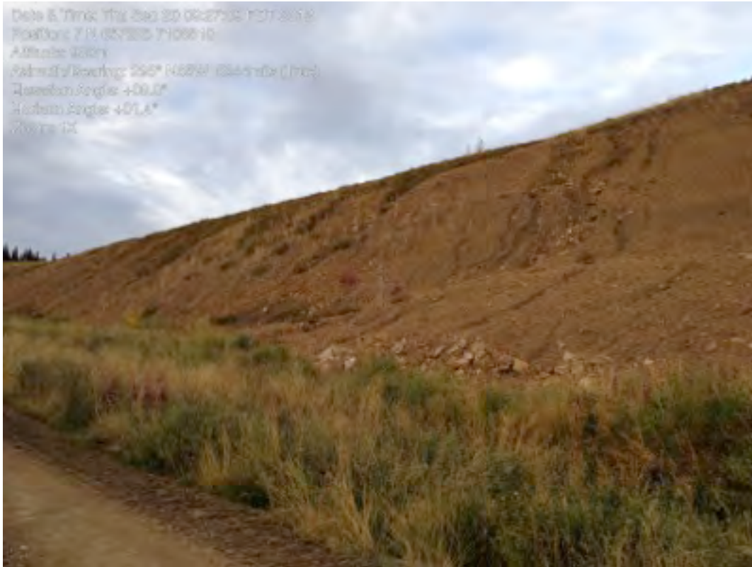
Plate 25: Erosion NW Corner North Golden Waste Dump
