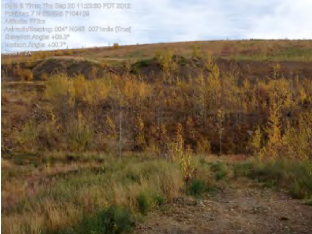
Plate 34: Breach in Heap Leach Containment Dyke above Pregnant Pond
