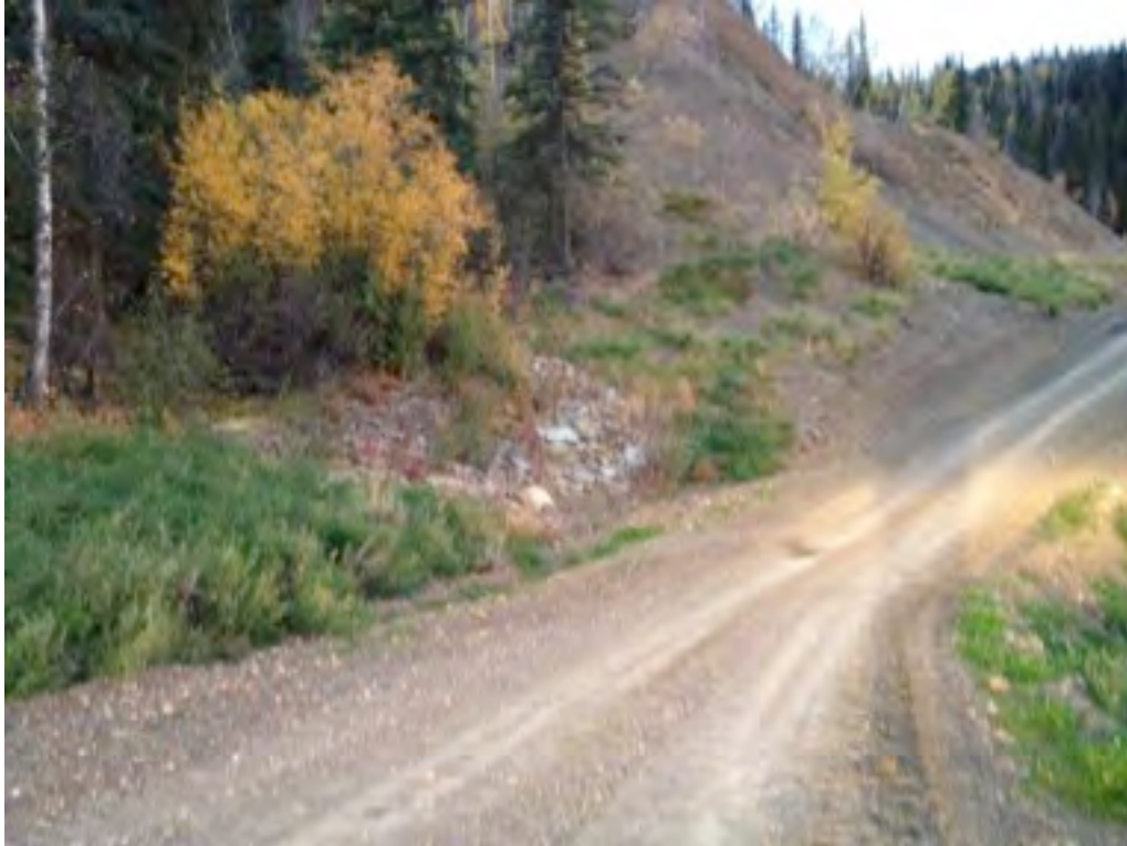
Plate 3: Haul Road Swale KP 1.2
