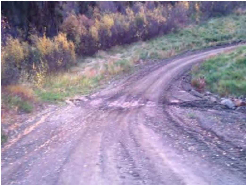
Plate 6: Haul Road Swale KP 1.8 - Repaired Washout
