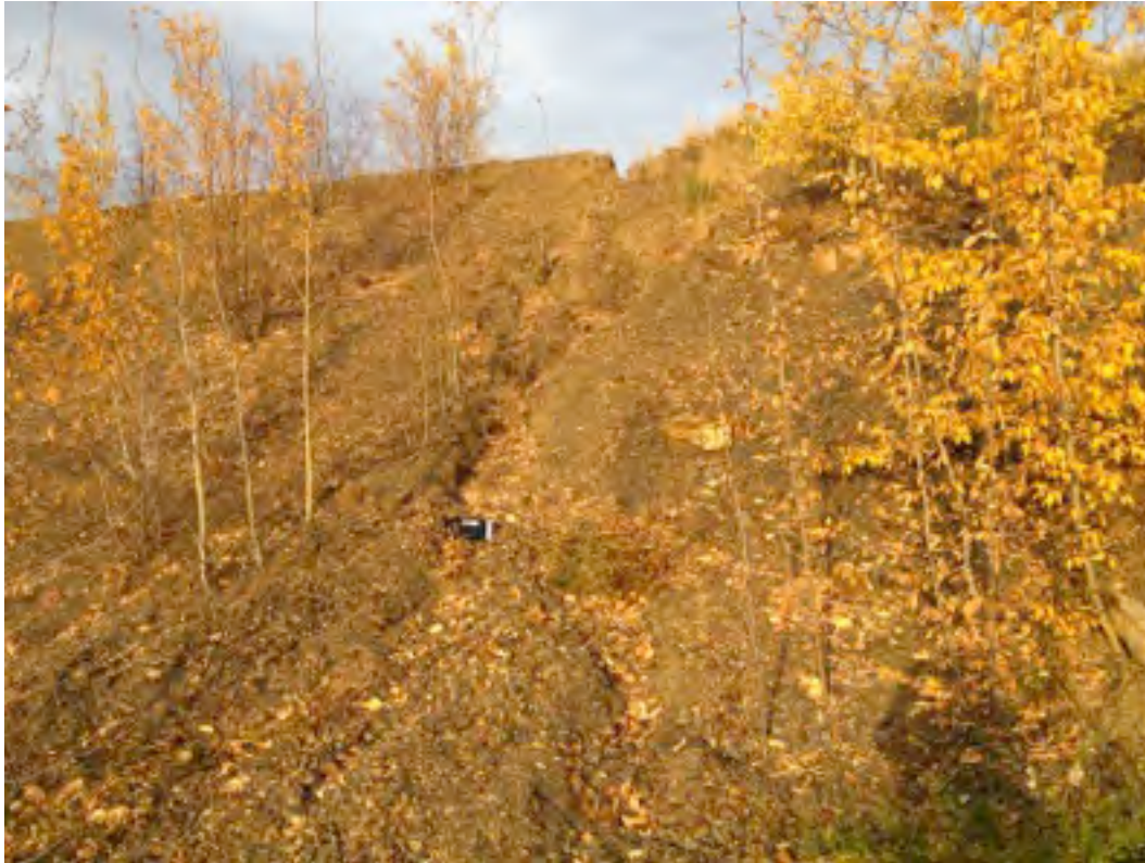
Plate 35: Erosion Channel North of Containment Dyke Breach
