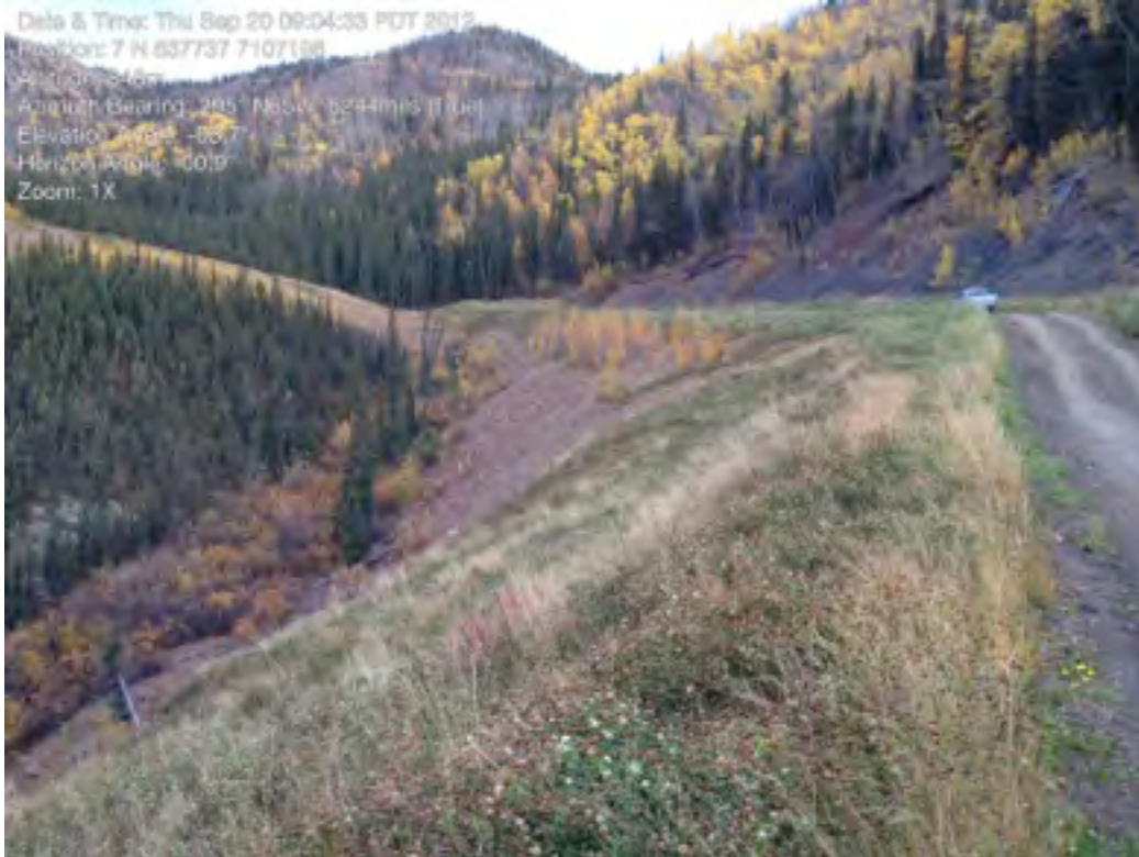
Plate 13: Lucky Haul Road Embankment
