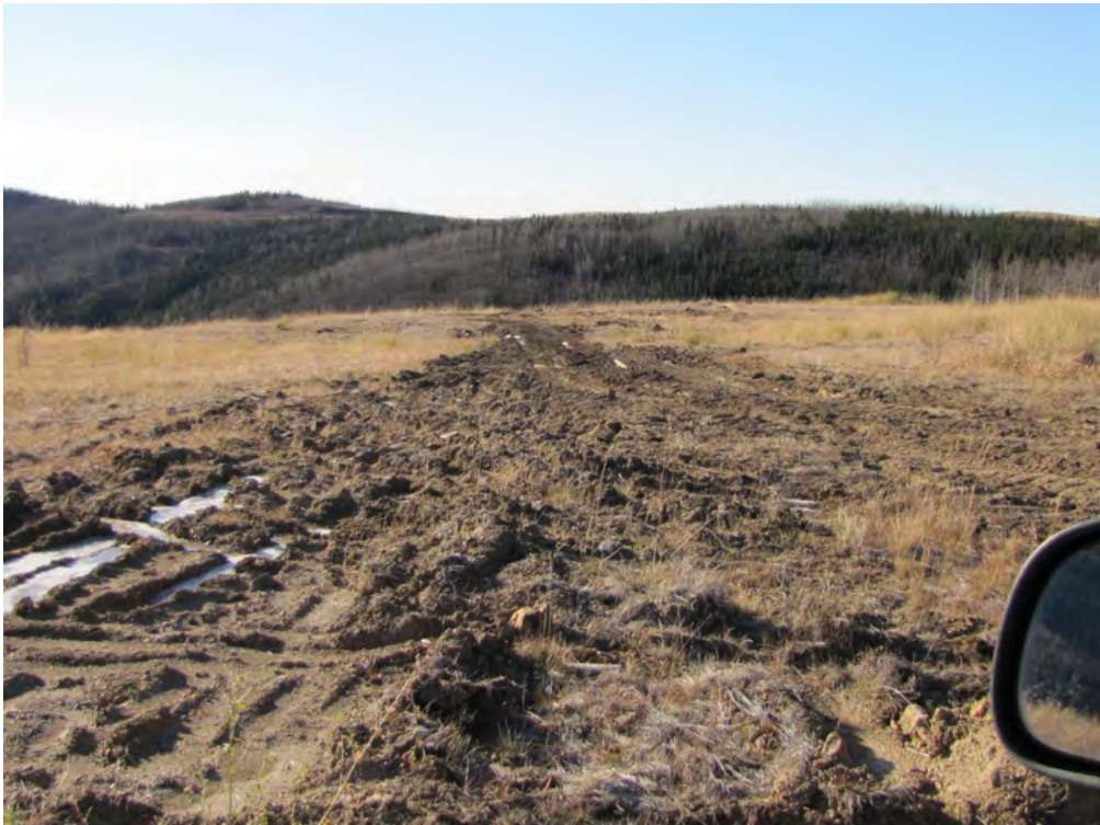
Vehicle tracks on cover of Blue waste rock dump.
