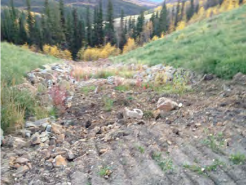
Plate 1: Haul Road Swale Discharge KP 0.6
