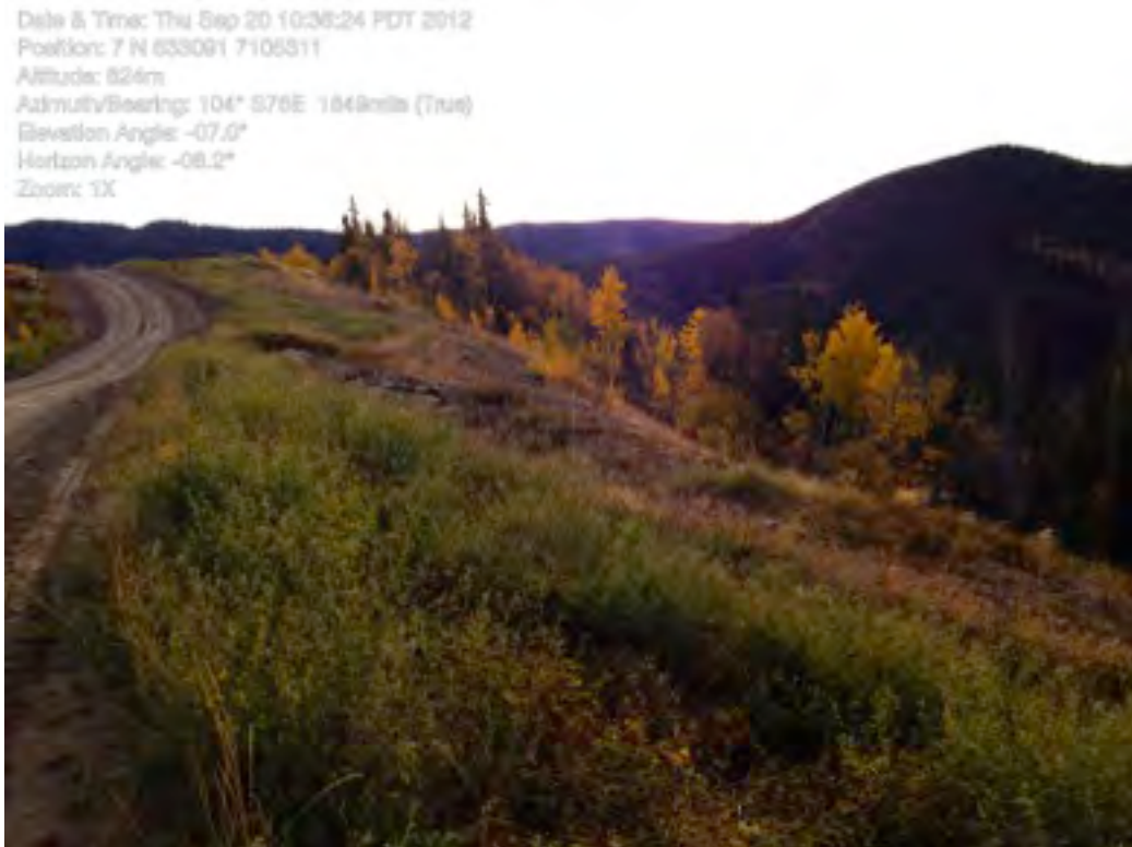
Plate 16: Pacific Pit Overflow Drainage Channel
