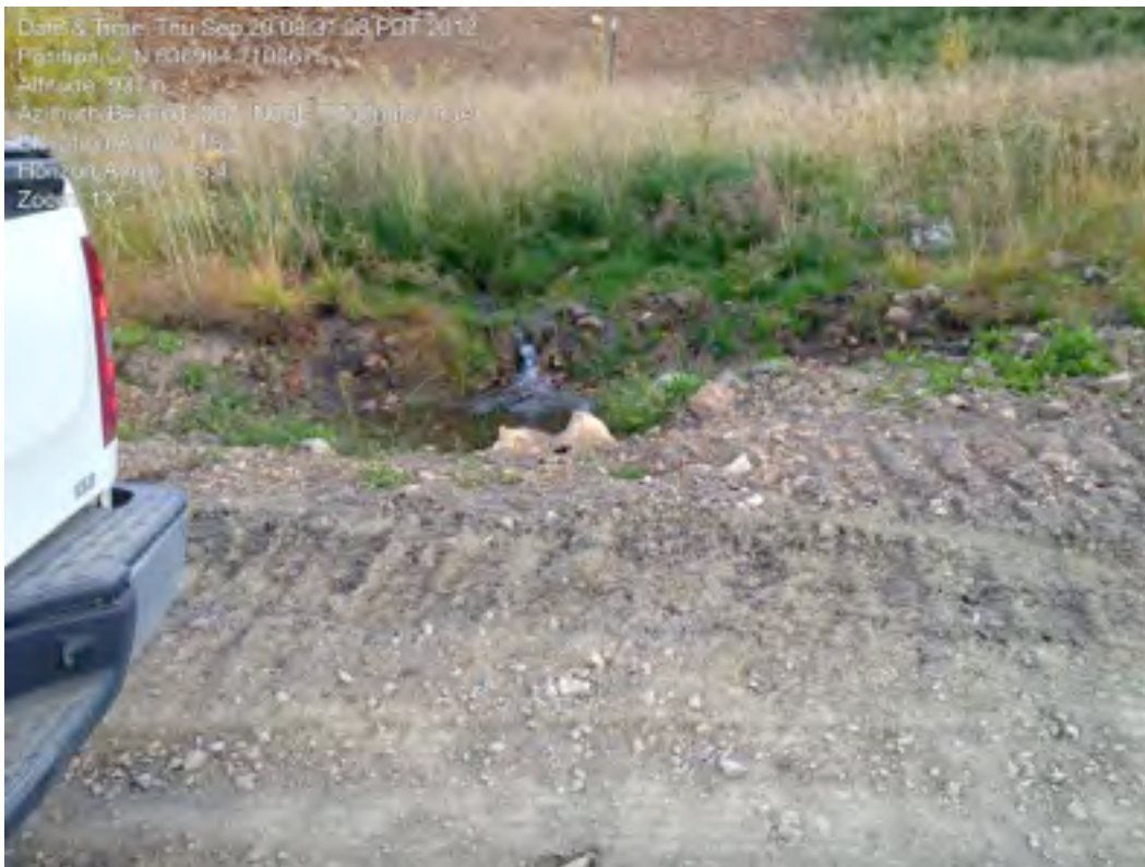
Plate 10: Haul Road Drainage KP 4.5 150mm HDPE Pipe
