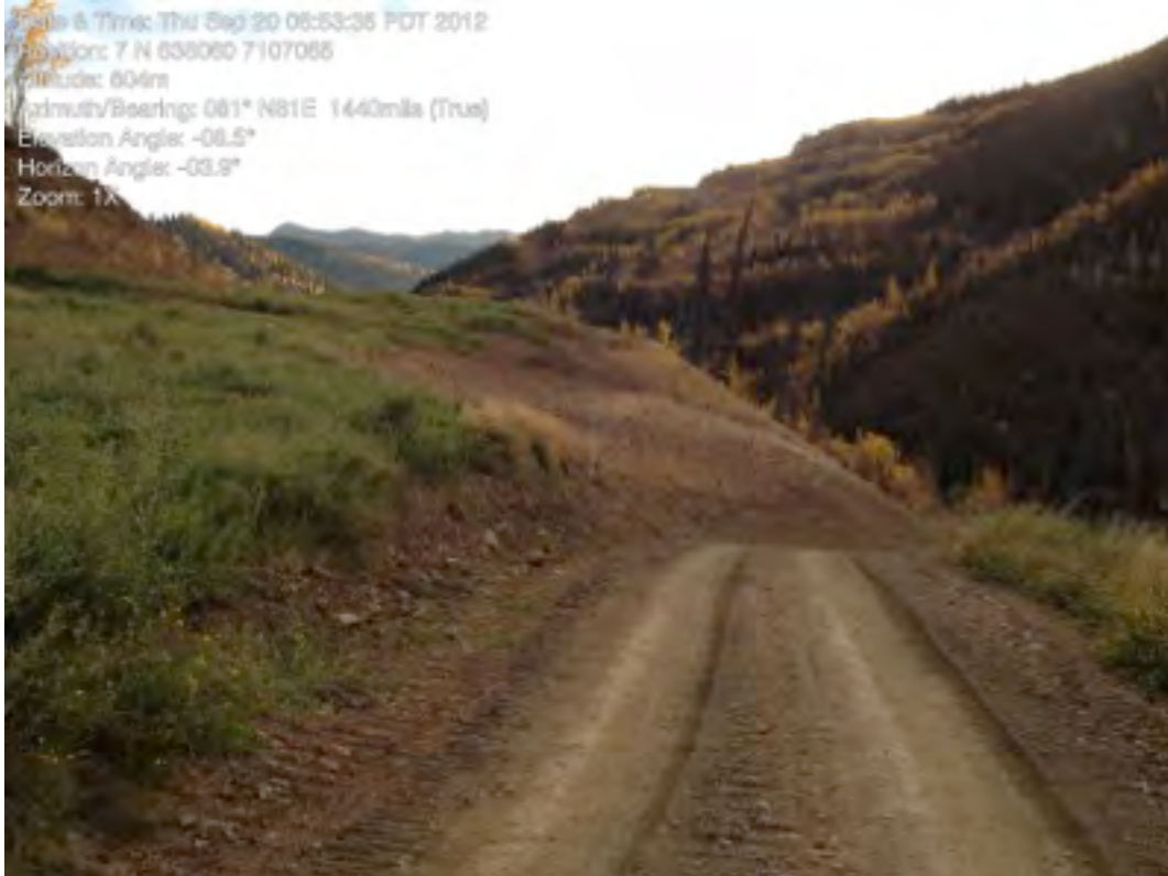
Plate 30: Bohemian Access Road Re-contoured Slump Area
