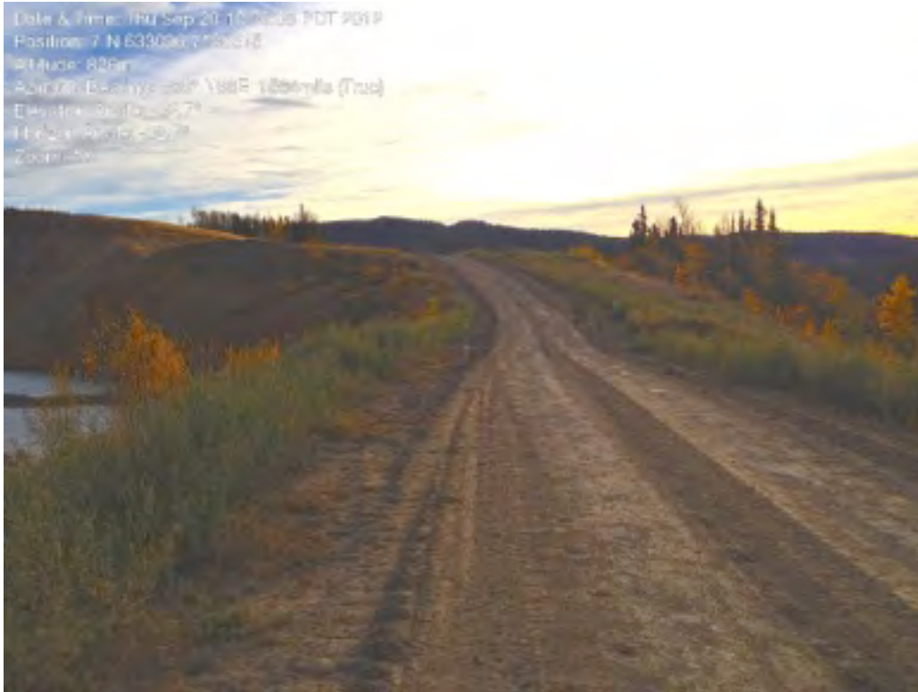
Plate 15: Sinkhole Repair at Pacific Pit Overflow
