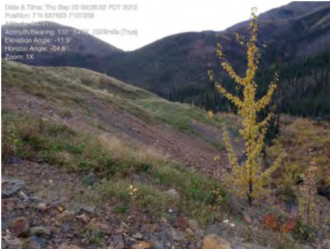
Plate 14: Embankment Stabilization Lucky Haul Road
