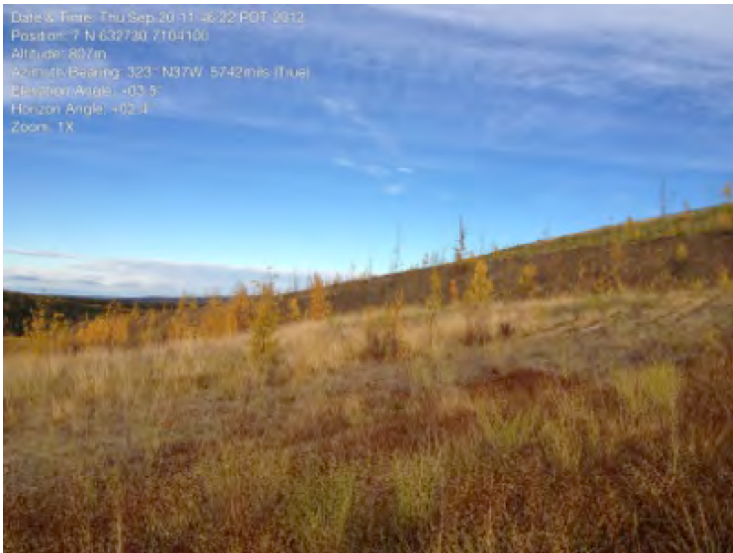
Plate 32: Heap Leach Containment Dyke Looking Northwest
