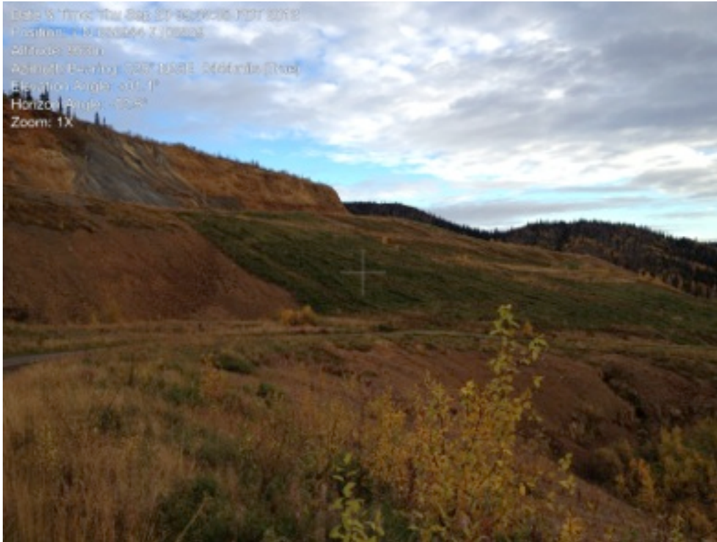
Plate 39: 2012 North Golden Reclaimed Waste Dump
