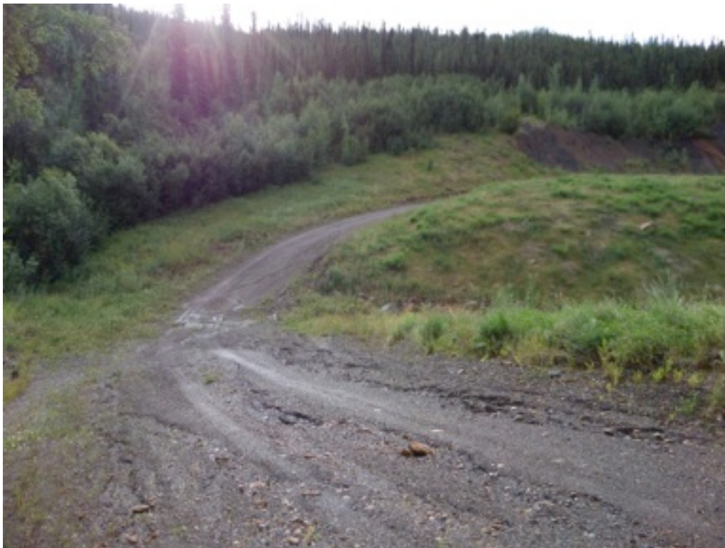
Plate 7: 2014 Haul Road 3.4 (Old KP 1.8) light surface rutting
