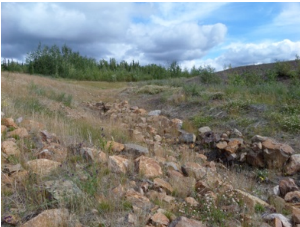
Plate 56: 2014 North Heap Leach Diversion Swale at Access Road
