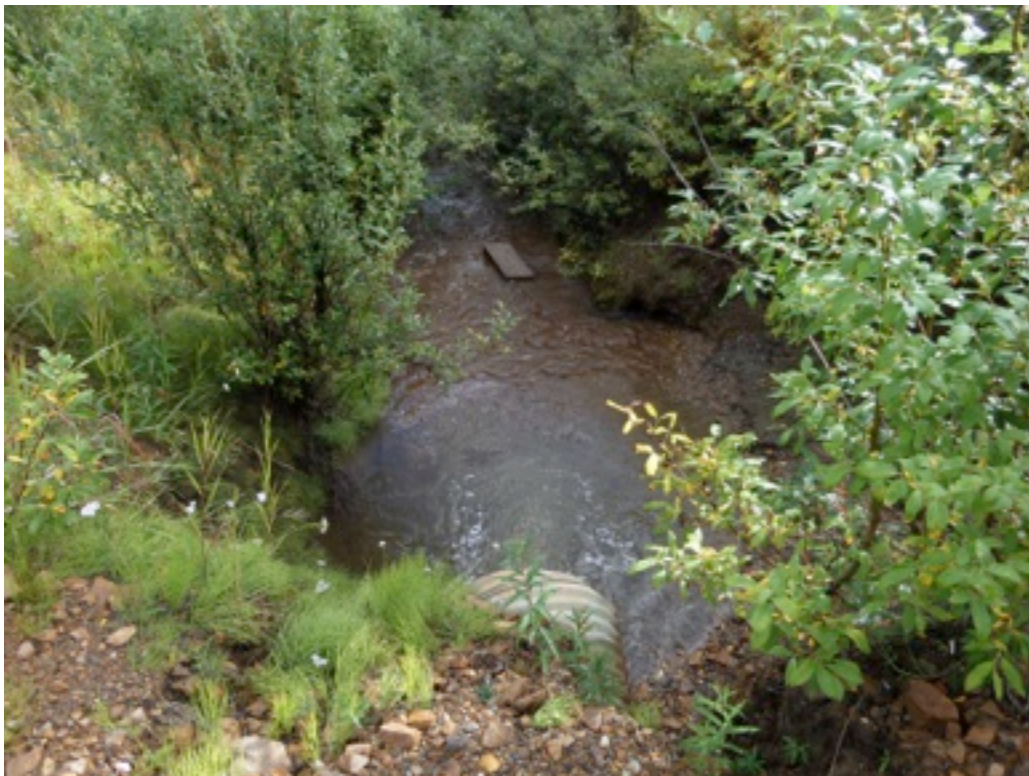
Plate 52: 2014 Bohemian Access Road 600mm Culvert
