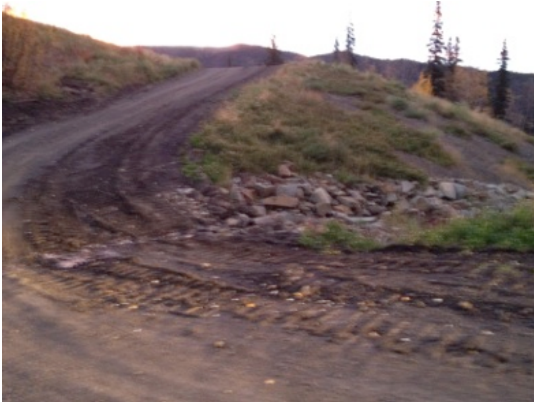
Plate 5: 2012 Haul Road Swale Discharge KP 3.1 (Old KP 1.5)
