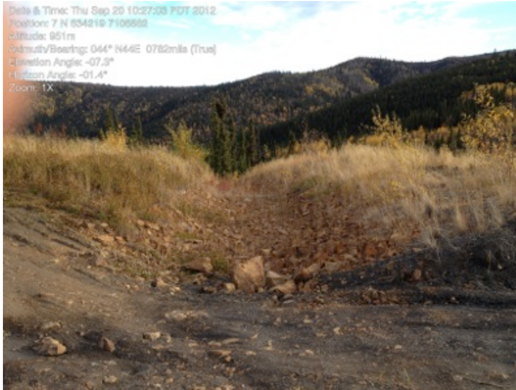
Plate 33: 2012 Moosehead Pit Overflow Channel
