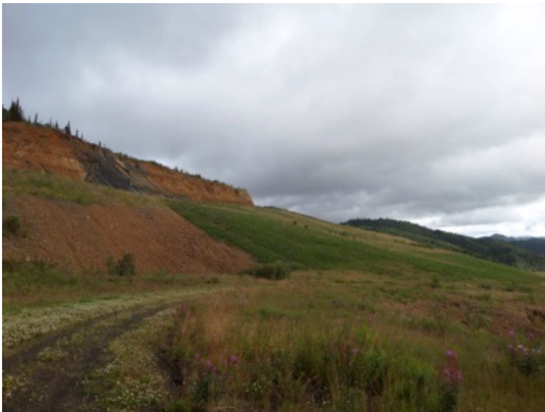
Plate 40: 2014 North Golden Reclaimed Waste Dump
