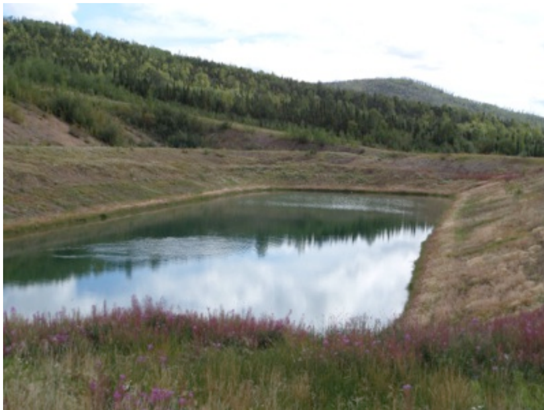
Plate 66: 2014 Overflow Pond Looking South - Overflow Weir Mid Berm
