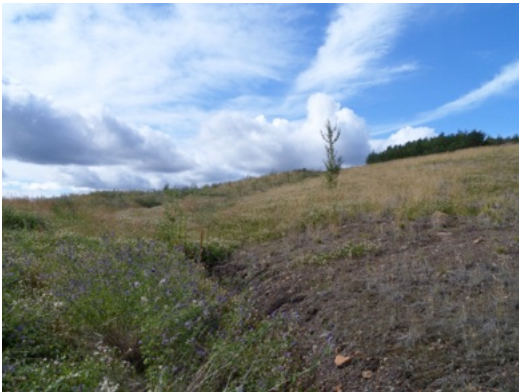
Plate 28: 2014 Erosion Channel Appears to Have Stabilized
