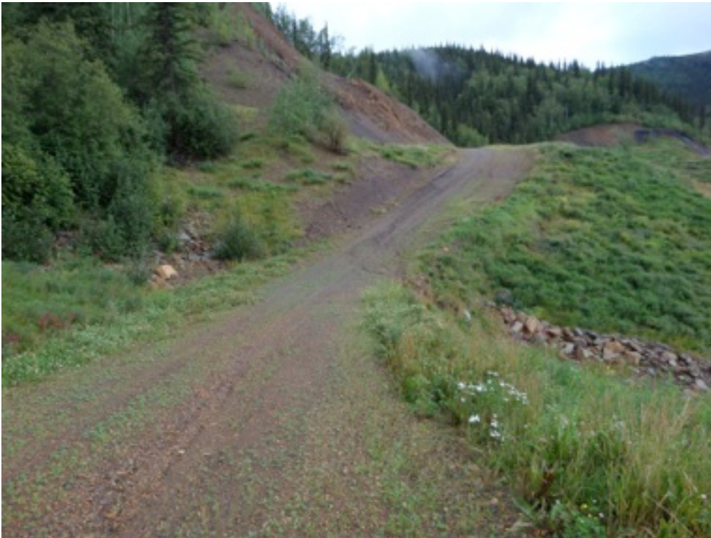
Plate 4: 2014 Haul Road Swale KP 2.8 (KP 1.2 Old Markers)
