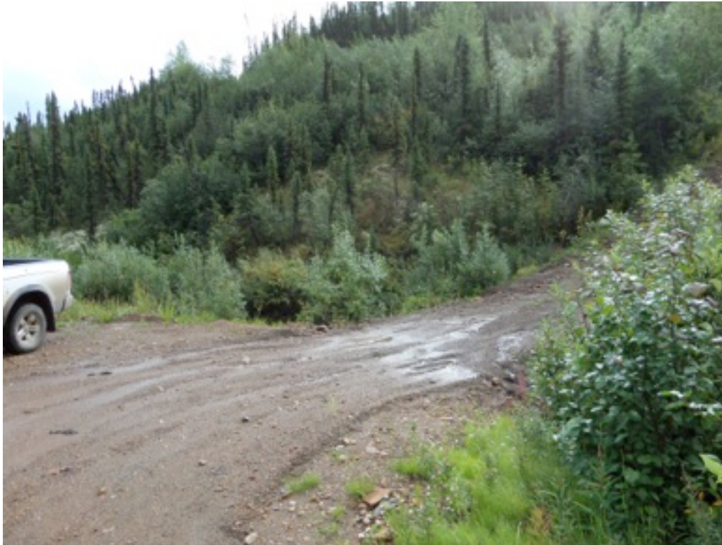
Plate 51: 2014 Bohemian Access Road Creek Crossing
