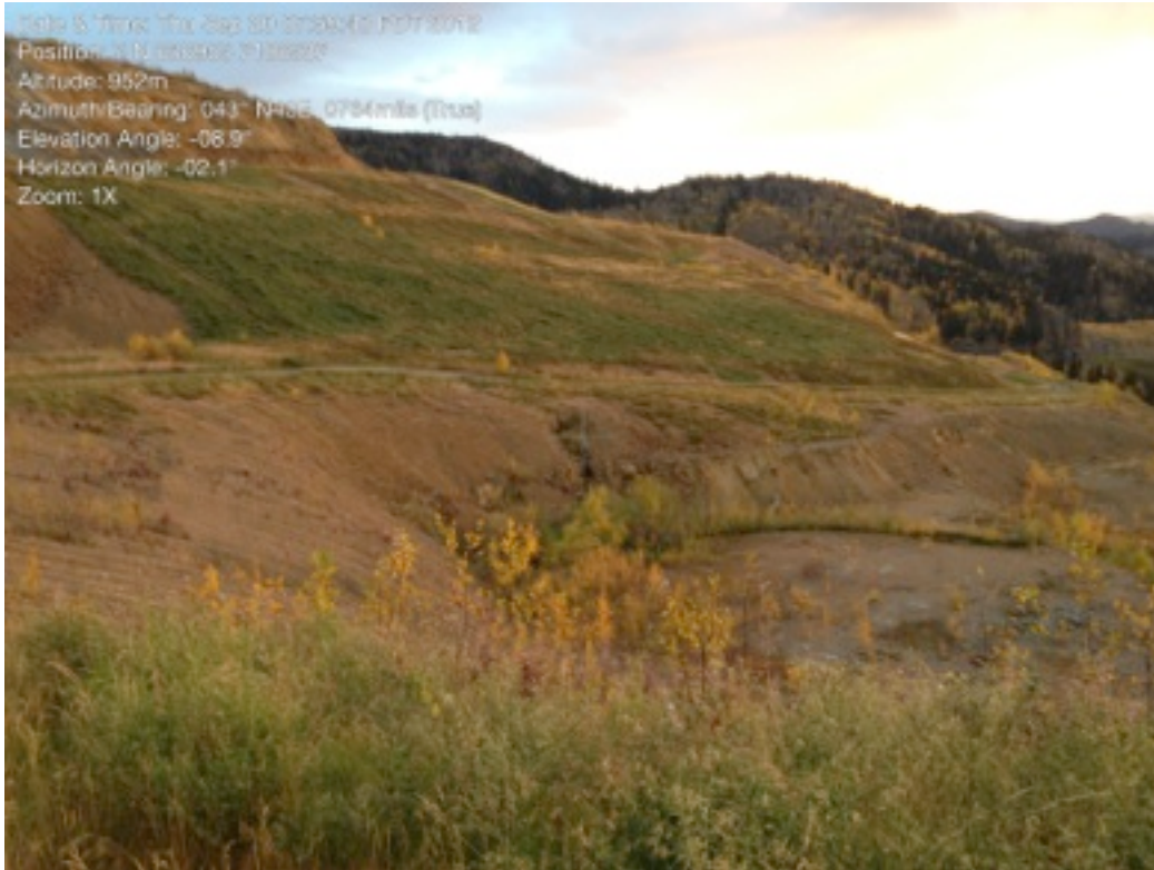
Plate 12: 2012 Haul Road Drainage KP 6.3 (Old KP 4.5) From Upper Fosters
