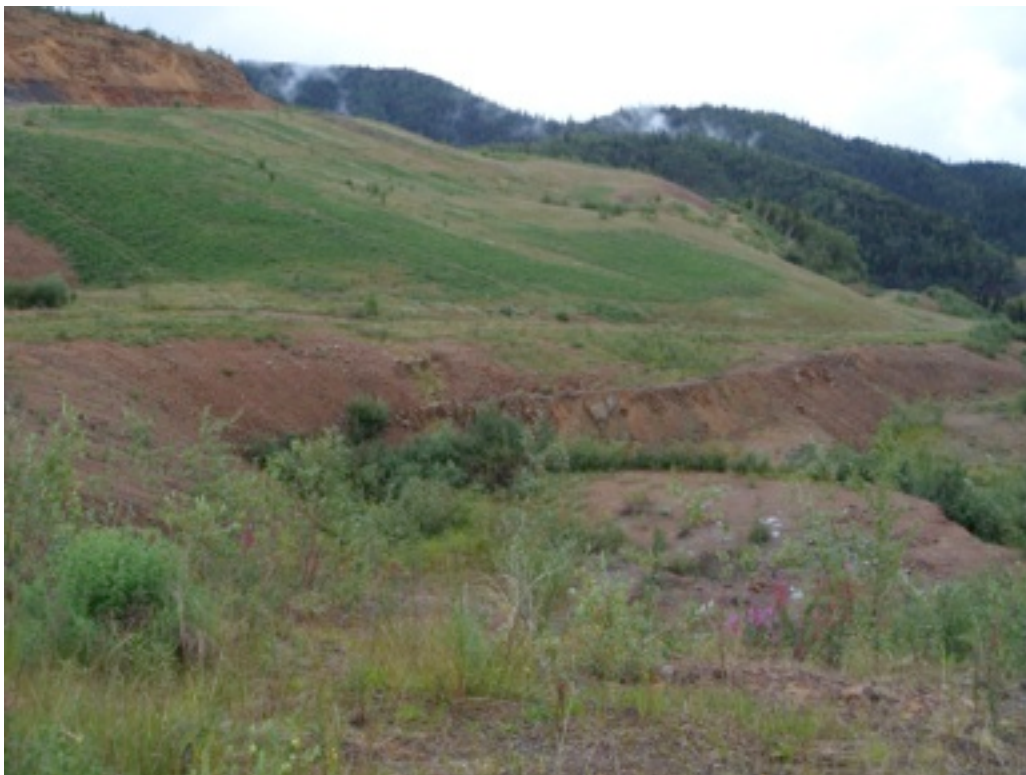
Plate 13: 2014 Haul Road KP 6.3 Showing Riprap Repairs
