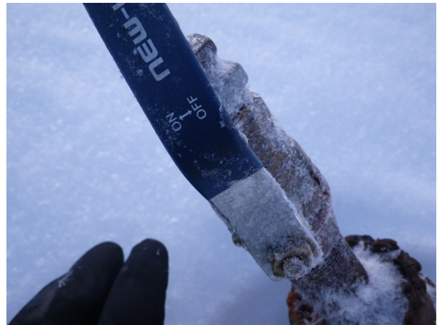
Photo 8: LF-XX-03 valve on and frozen.
