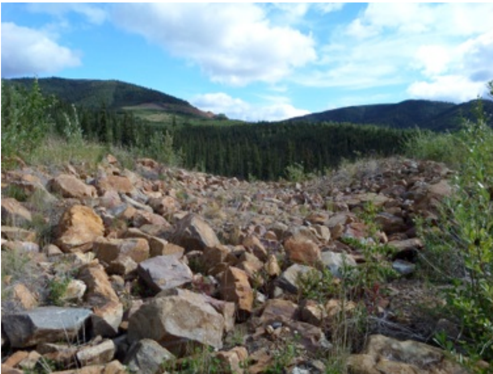
Plate 30: 2014 Blue Pit Overflow Channel
