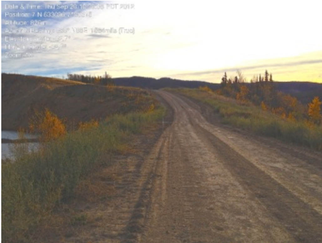
Plate 21: 2012 Haul Road Sinkhole Repair at Pacific Pit Overflow
