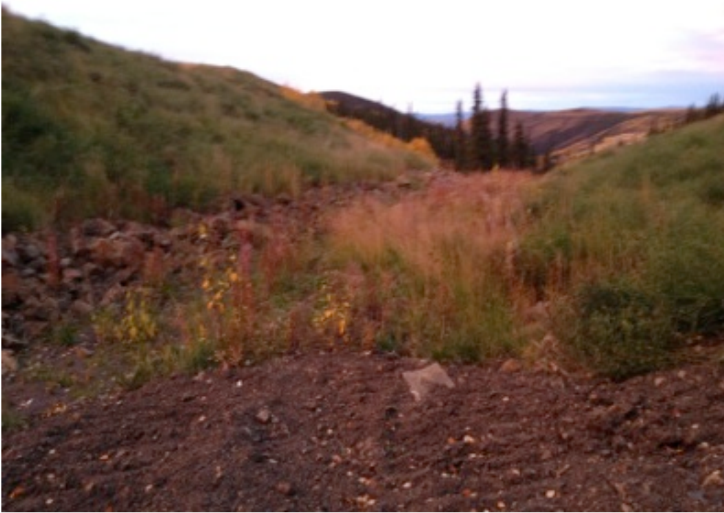
Plate 8: 2012 Haul Road Swale KP 3.4 (Old KP 1.8) - Repaired Washout
