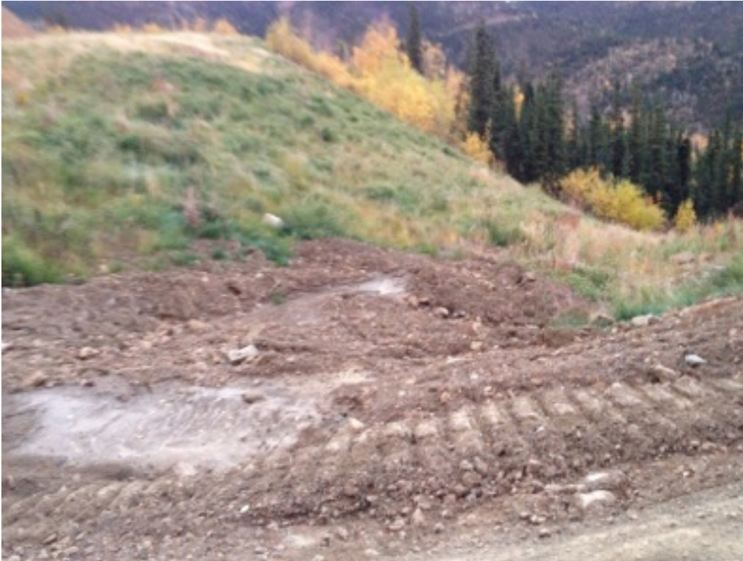
Plate 10: 2012 Haul Road Swale KP 4.7 (Old KP 3.2) - Repaired Washout
