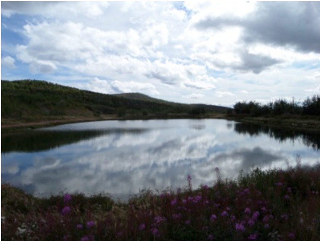
Plate 64: 2014 Barren Pond Looking South - Overflow Spillway on Left
