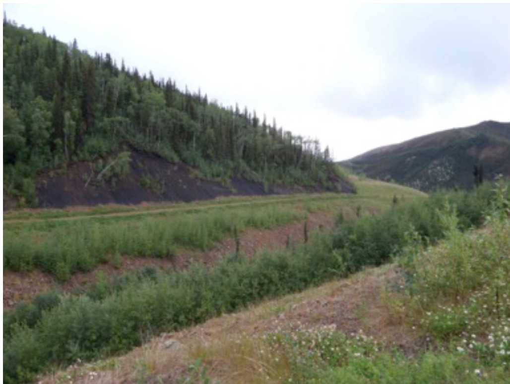
Plate: 20 2014 Lucky Haul Road Embankment Stabilization
