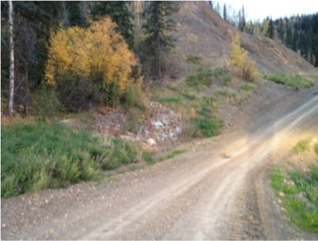
Plate 3: 2012 Haul Road Swale KP 2.8 (KP 1.2 Old Markers)
