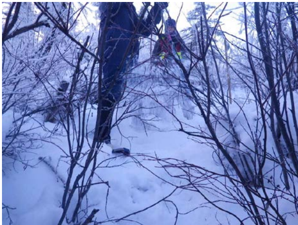
Photo 7: BC-2, looking upstream from below weir, lots of overflow ice
