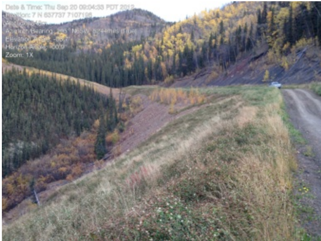
Plate 19: 2012 Lucky Haul Road Embankment Stabilization
