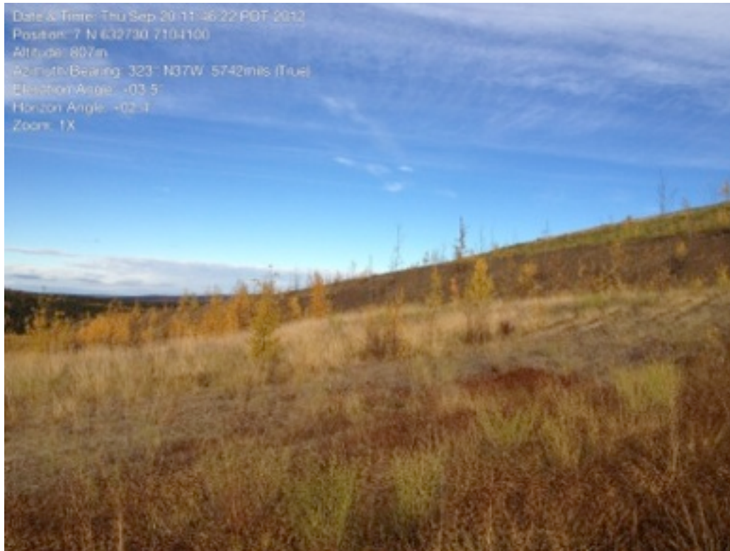
Plate 57: 2012 Heap Leach Containment Dyke Looking Northwest
