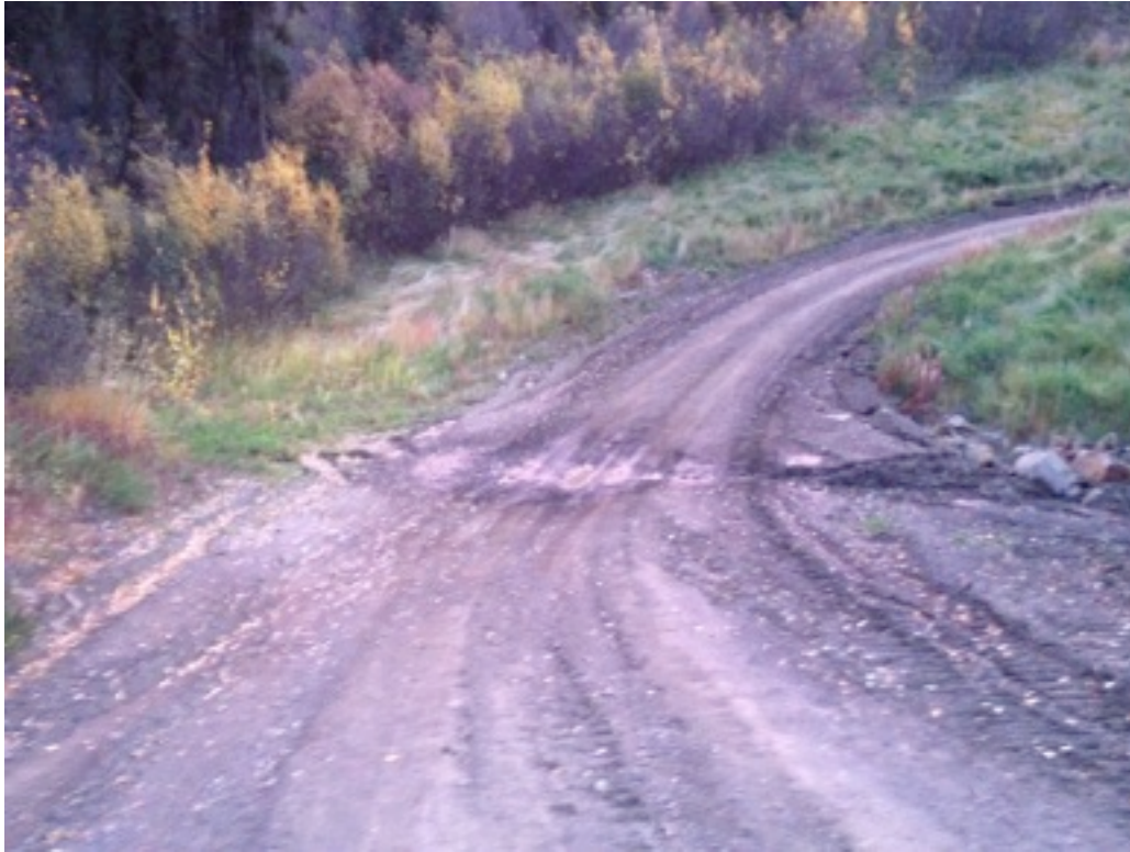
Plate 6: 2012 Haul Road Swale KP 3.4 (Old KP 1.8) - Repaired Washout
