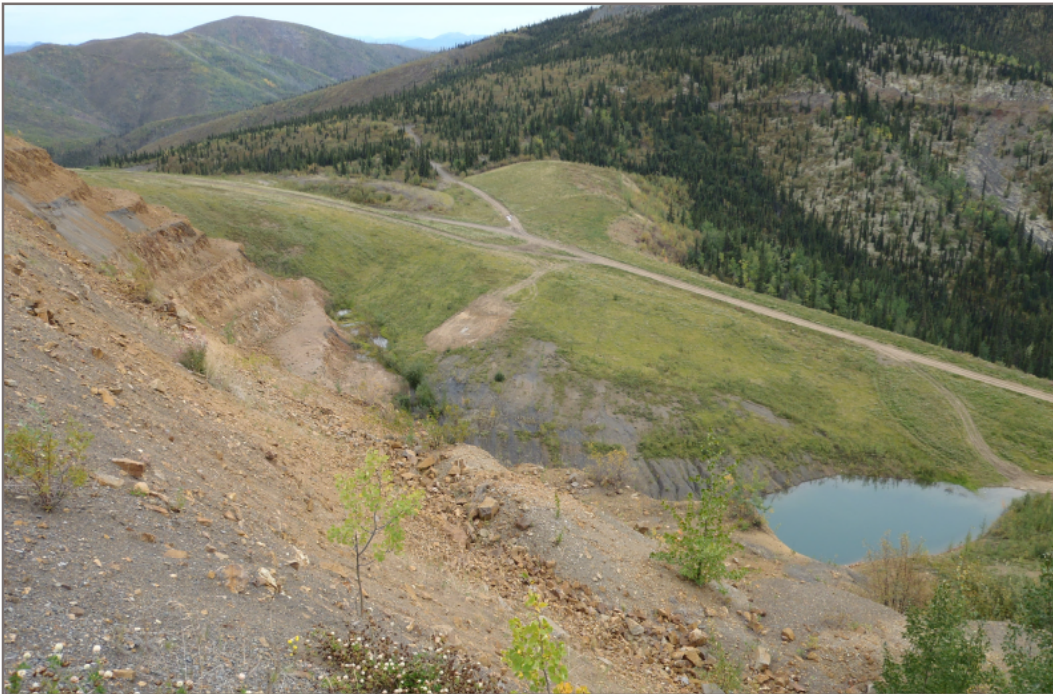
Photo 14: Kokanee Stable pit walls and waste rock dumps Facing east — August 23, 2016
