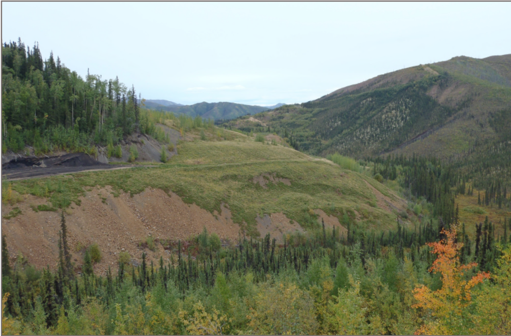
Photo 5: Primary Haul Road Historic instability near Lucky Pit Facing northeast — August 23, 2016
