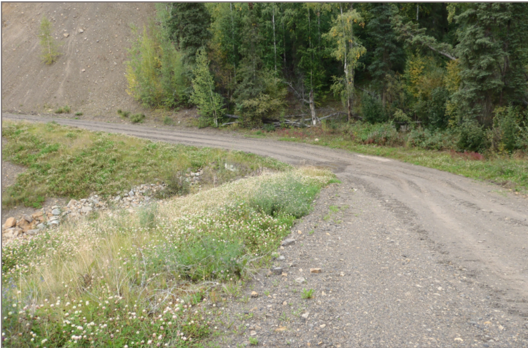
Photo 2: Primary Haul Road Drainage Crossing #3 Facing northwest — August 23, 2016
