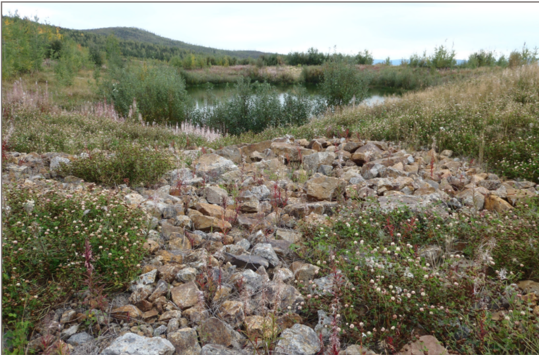
Photo 12: Process Ponds Pregnant Pond armoured emergency spillway Facing south — August 23, 2016
