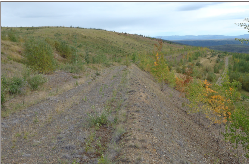
Photo 8: Containment Dyke Stable heap leach containment dyke Facing east — August 23, 2016
