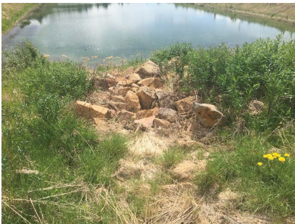
Photo 3: Dry overflow channel into Pond 3, BC-28B
