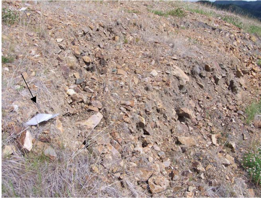
Plate 1: Slumped bank in area of Lucky road (note: clipboard for scale)
