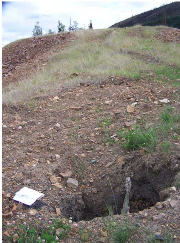
Plate 2: Sinkhole atop Lucky open pit
