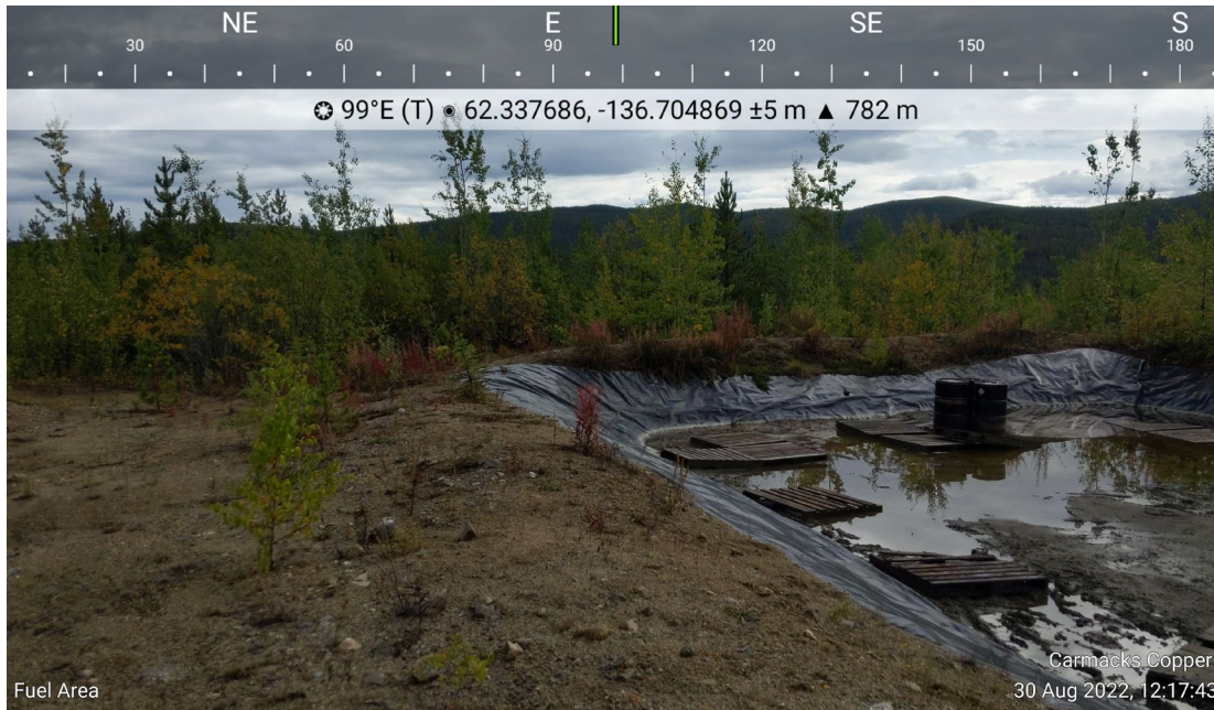
Photo 9: Water accumulation in fuel bund
