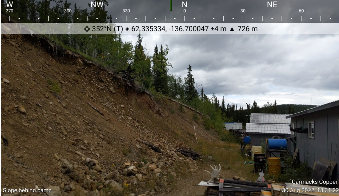
Photo 2: Slope behind camp – slope is in satisfactory condition
