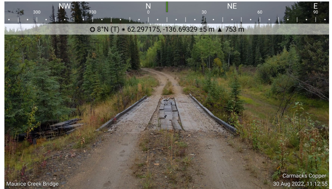
Photo 22: South abutment of Merrice Creek bridge
