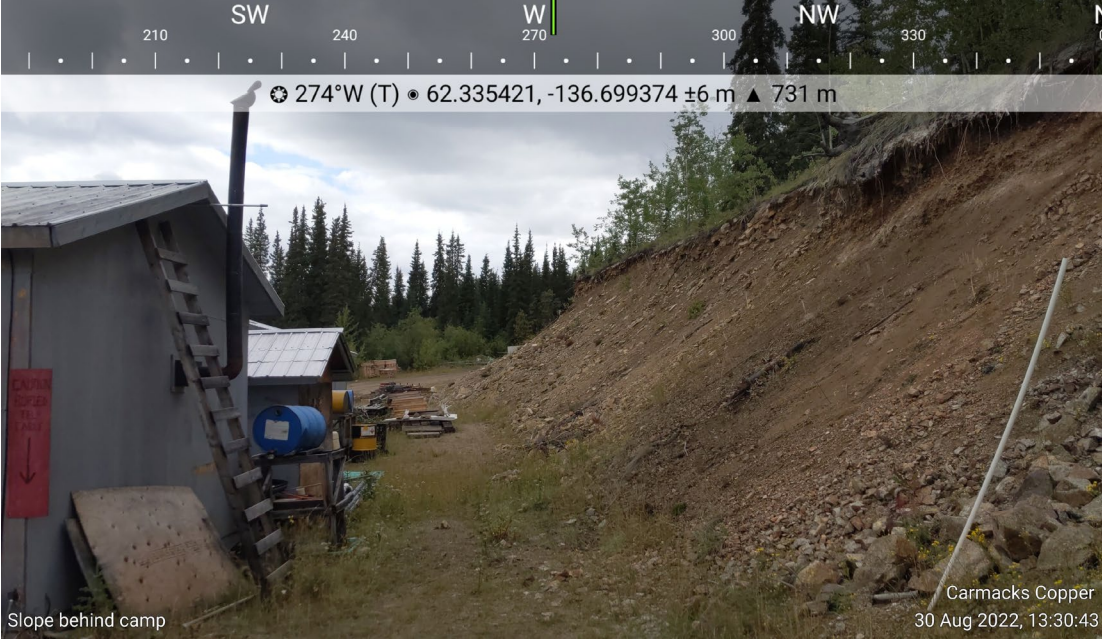
Photo 1: Slope behind camp – slope is in satisfactory condition
