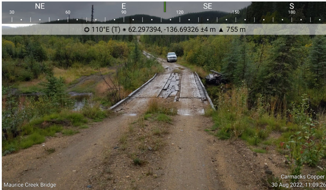
Photo 21: North abutment of Merrice Creek bridge
