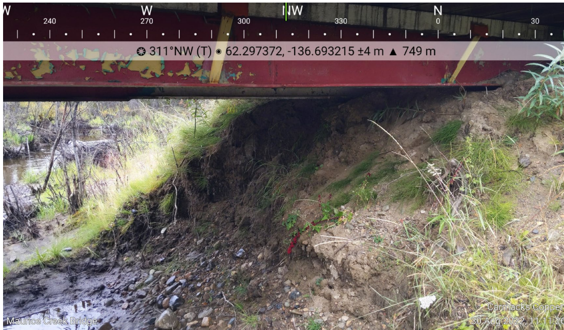
Photo 19: North abutment of Merrice Creek bridge
