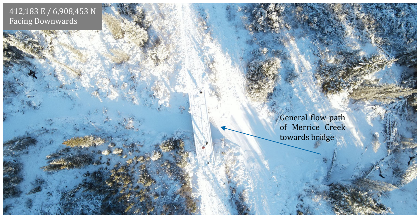
Photo 15: Aerial view of Merrice Creek bridge
