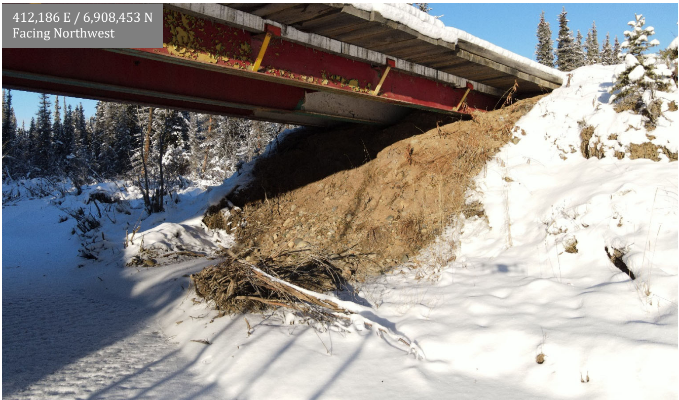
Photo 13: Merrice Creek bridge north abutment
