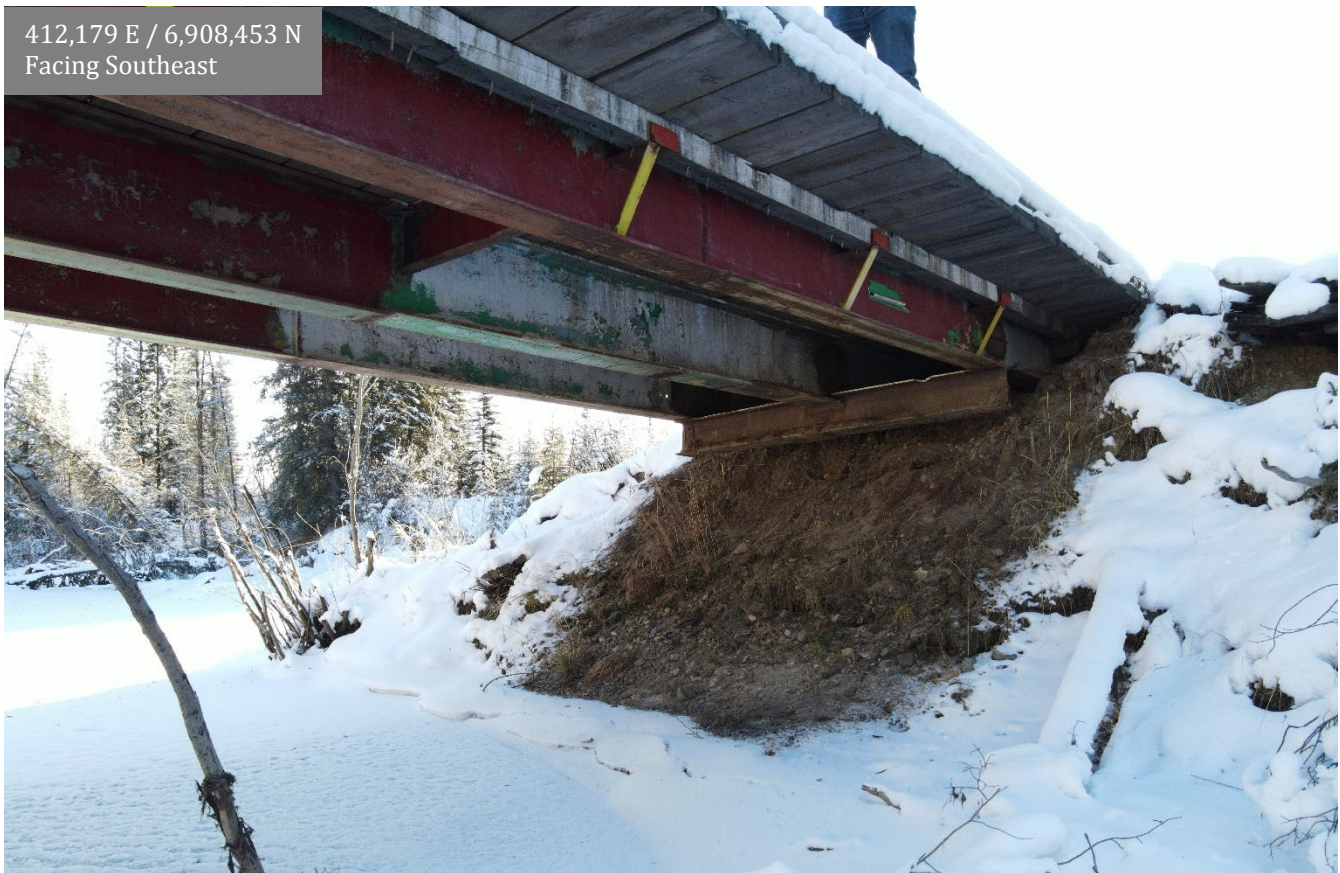
Photo 14: Merrice Creek bridge south abutment
